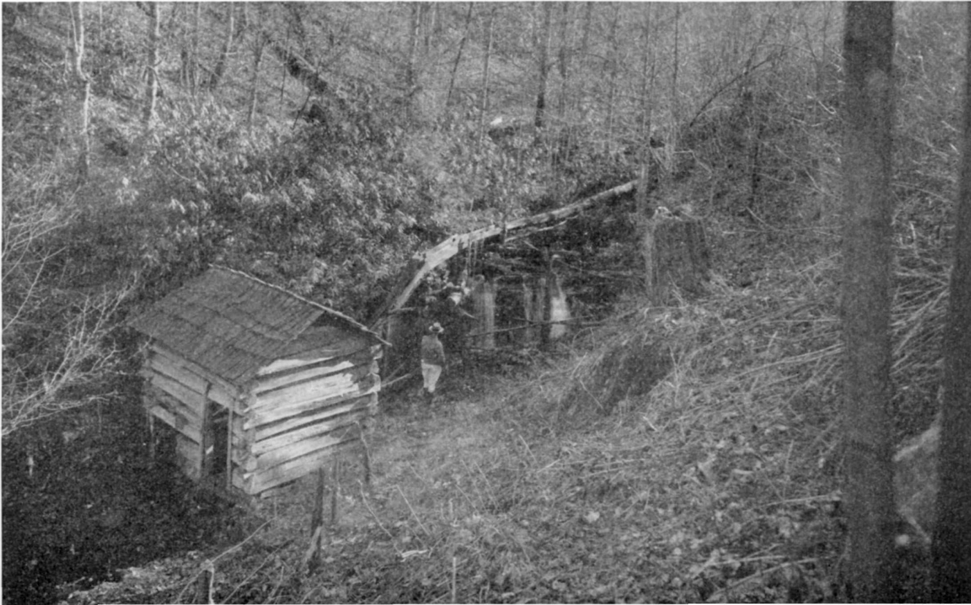
A tub mill on the Ashley Rayfield Place, Injun Creek, Greenbrier, Tenn. These small mills are usually found in the more rugged and isolated sections of the mountains. Constructed purely for domestic use, the building was simple, and its operation was well adapted to the small, rapid-falling mountain streams
