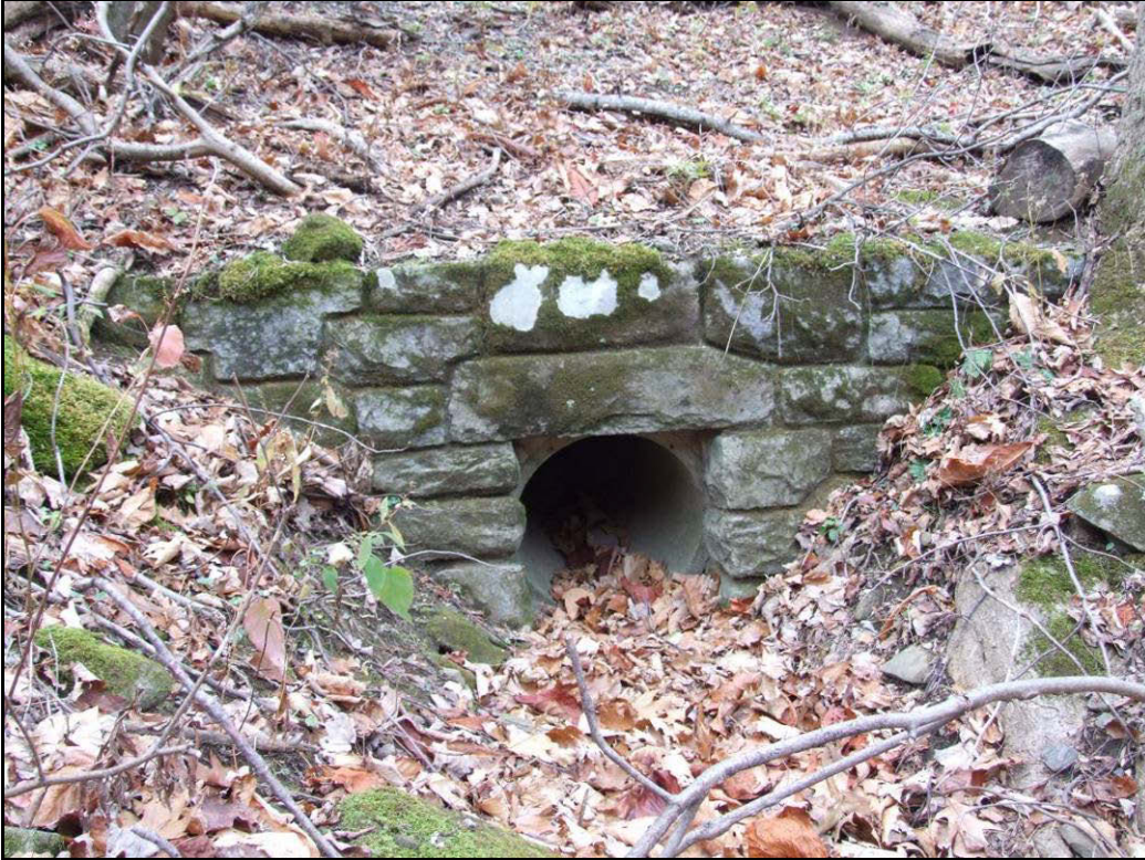
Figure 33. Pipe Culvert with Stone Masonry Faced Headwall, Milepost 3 (No. 46).
