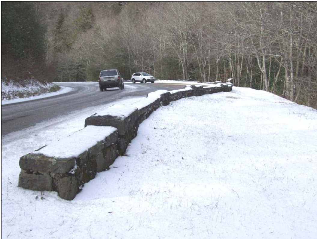
Figure 51. Parking Area with Crenellated Masonry Guard Wall (No. 156, Mile 10).
