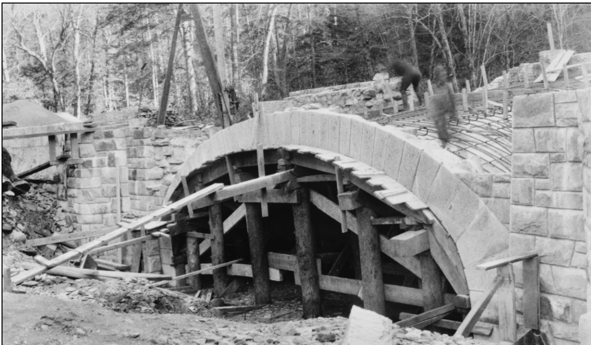
Figure 3. Masonry Arch Under Construction, 1935 (E.E. Exline, Photographer, GRSM Archives).
