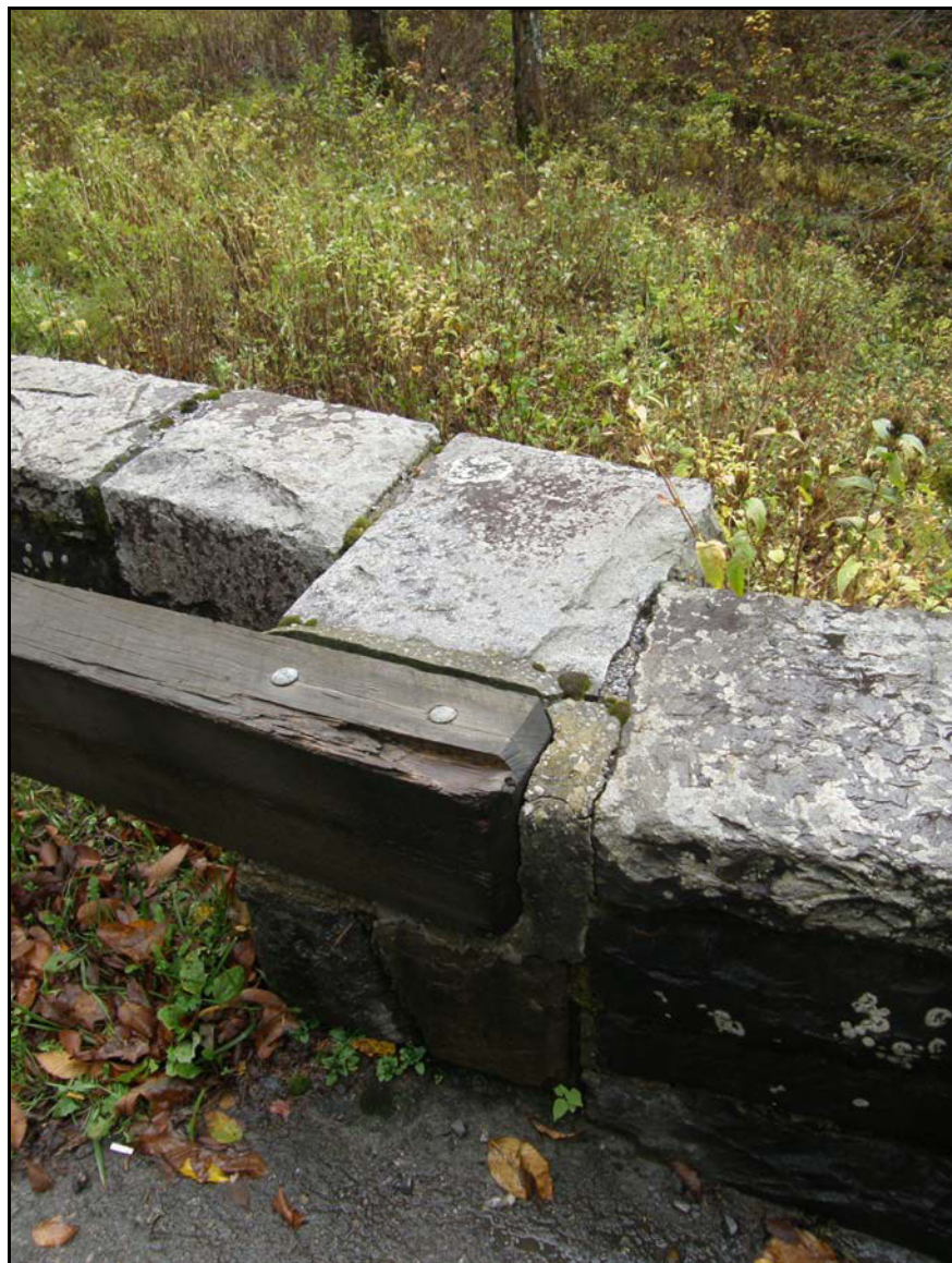
Figure 44 Timber Guardrail Attached to Stone Masonry Guard Wall.
