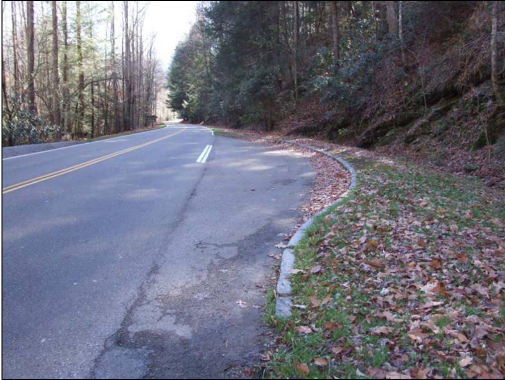
Figure 54. Pull Off with Stone Curbing (Number 13, Milepost 1)
