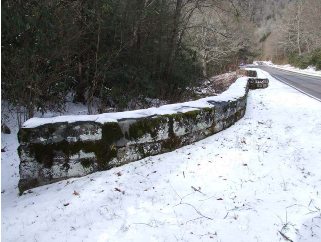
Figure 24. Walker Camp Prong Bridge Wing walls.
