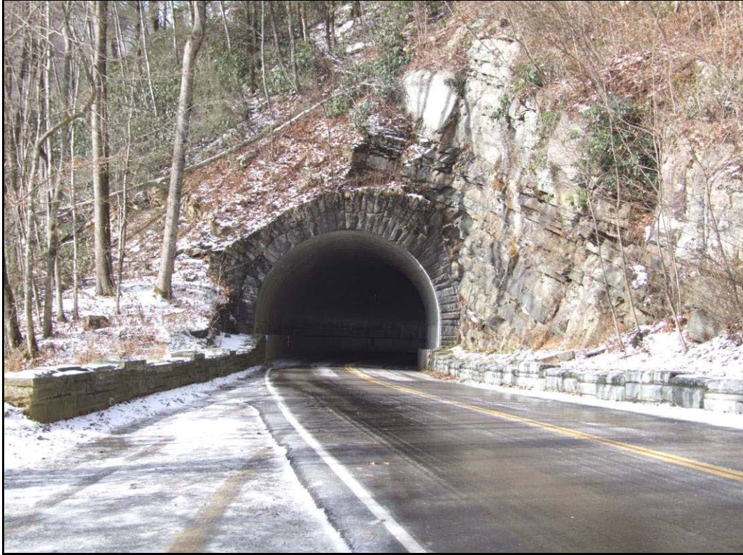
Figure 28. View of Chimney Tops Tunnel, South Portal.
