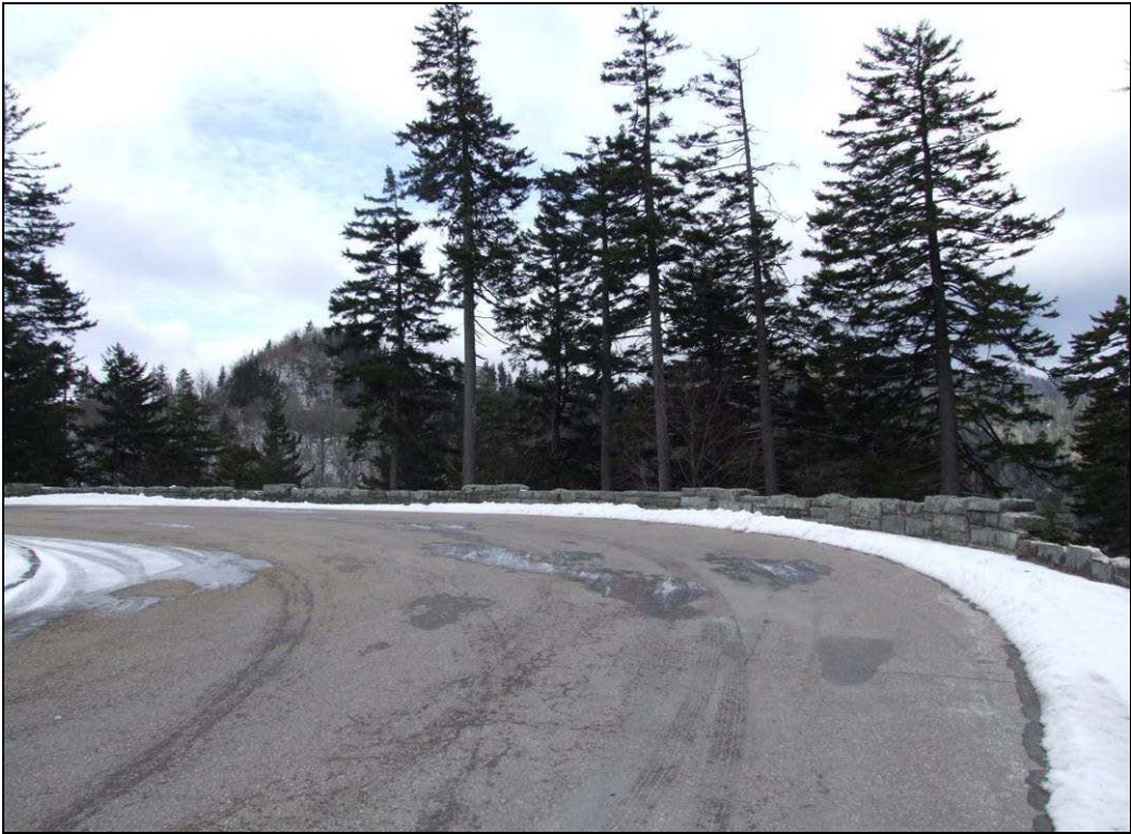
Figure 52. Overlook with Crenellated Masonry Guard Wall.
