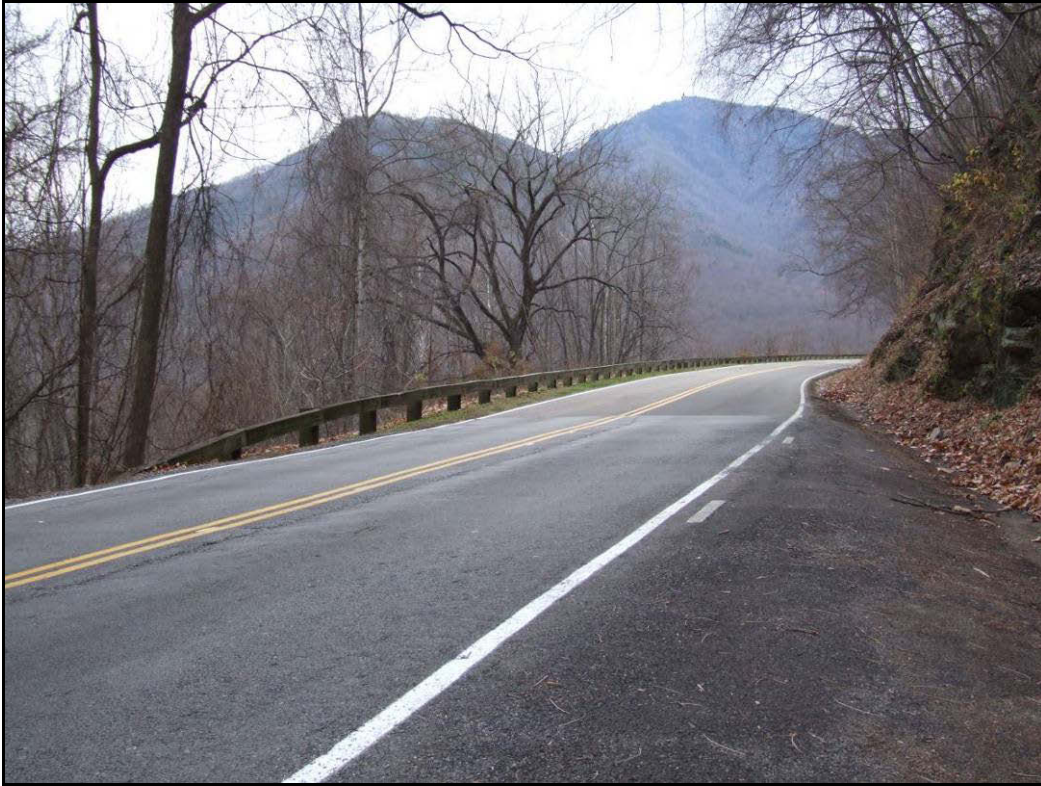
Figure 45. Steel Backed Timber Guardrail Along Newfound Gap Road.
