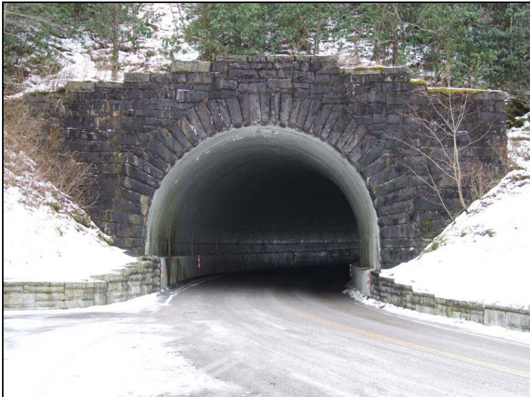
Figure 29. View of Morton Tunnel, North Portal.
