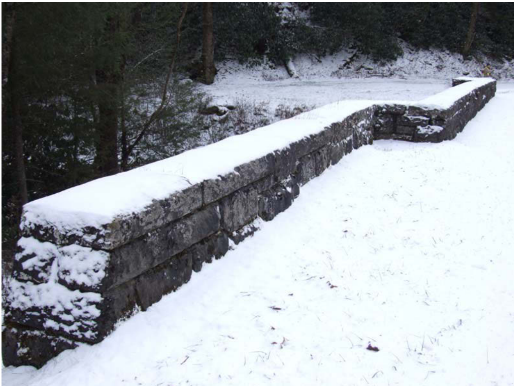
Figure 25. West Prong Little Pigeon River Bridge Wing Walls
