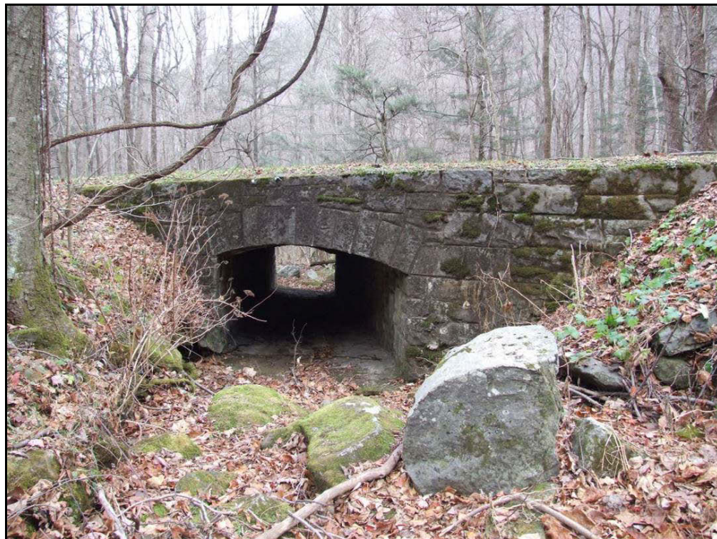
Figure 33. Large Box Culvert with Stone Masonry Faced Headwall, Milepost 5 (No. 73).
