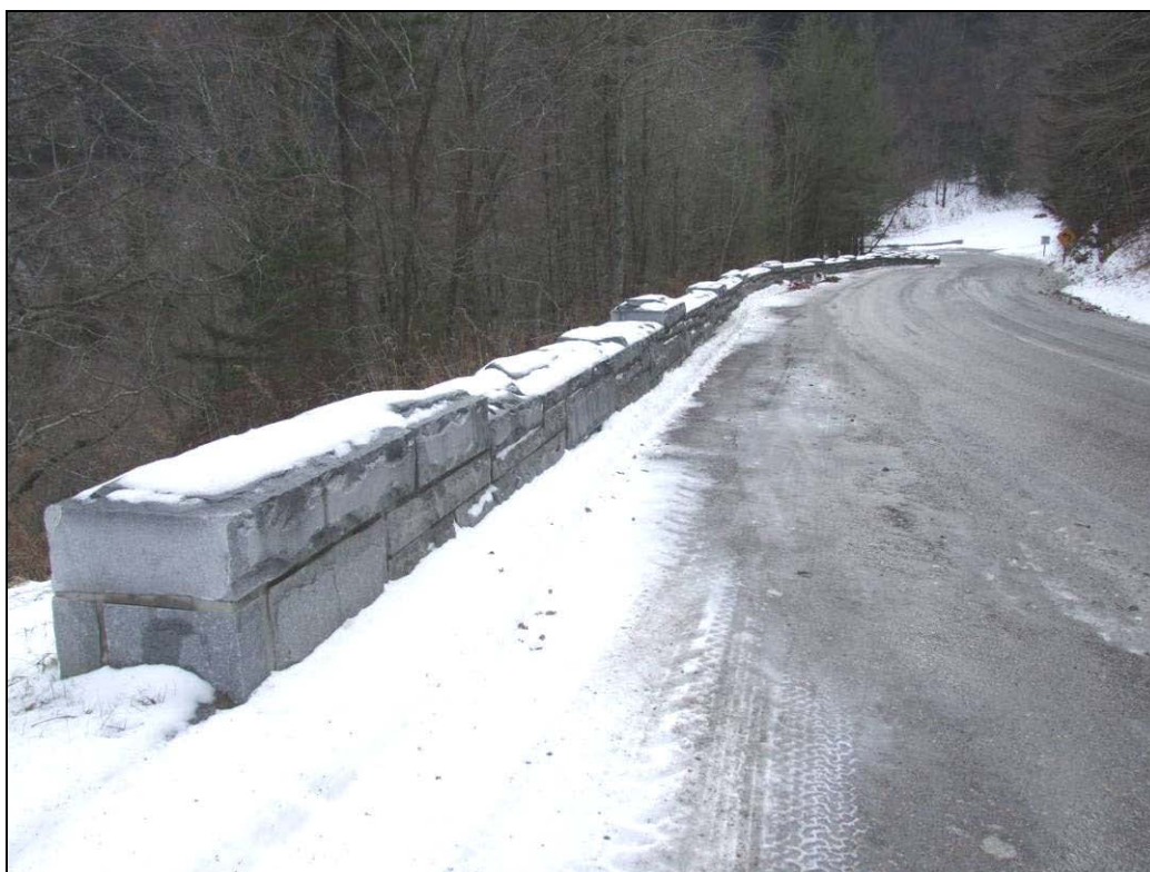
Figure 41. Guard Wall Built 2001-2000 Near Morton Tunnel (No. 216, Milepost 13)
