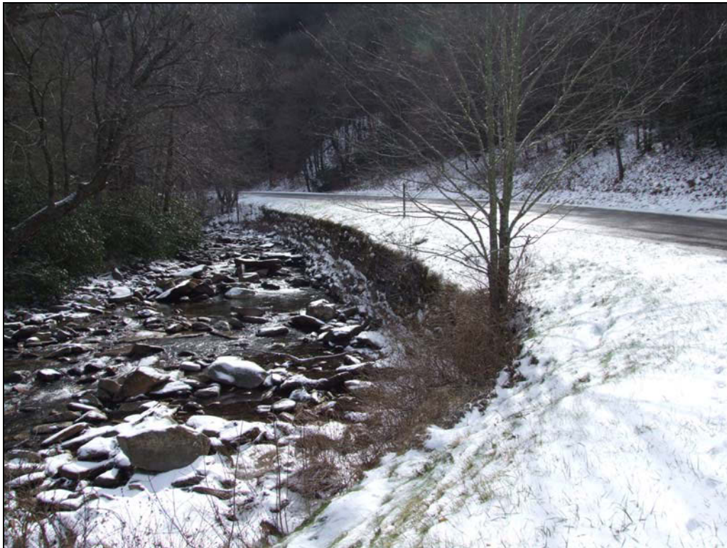
Figure 42. Stone Masonry Retaining Wall.
