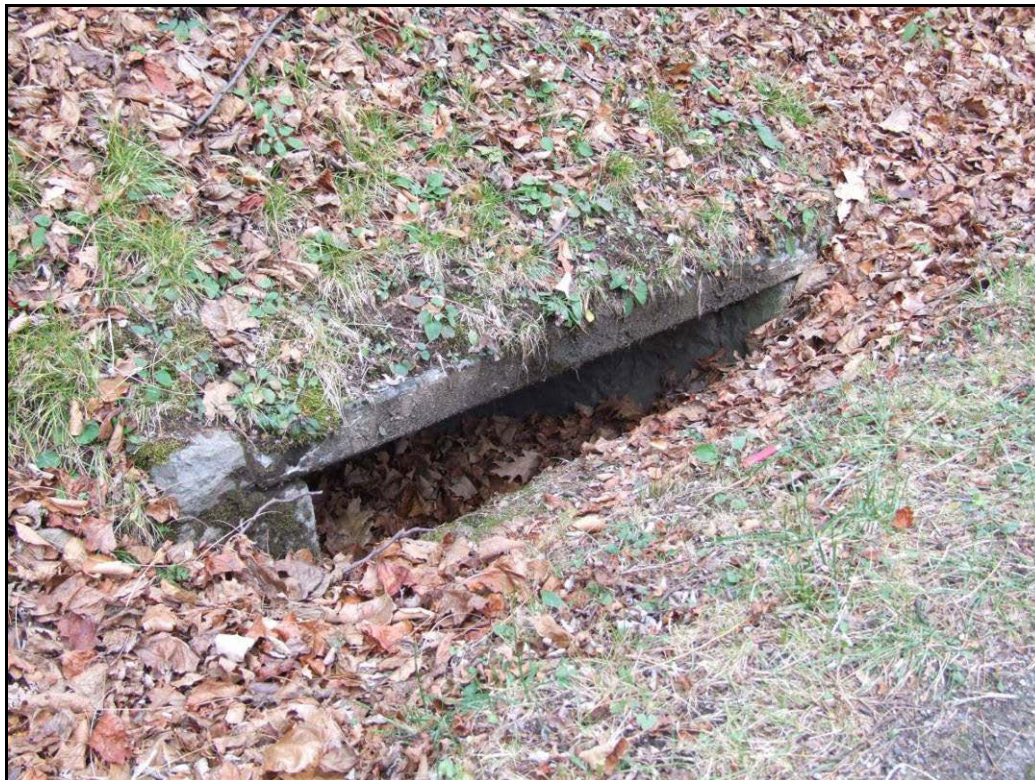
Figure 34. Drop Inlet Slab Culvert, Milepost 5 (No. 67).
