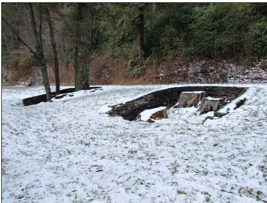
Figure 55. Tree Wells, Milepost 12 (No. 254).
