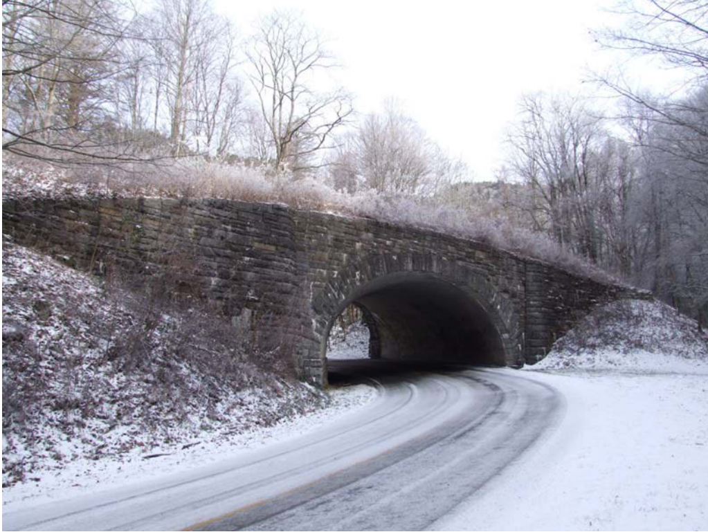
Figure 27. Loop Over Bridge.
