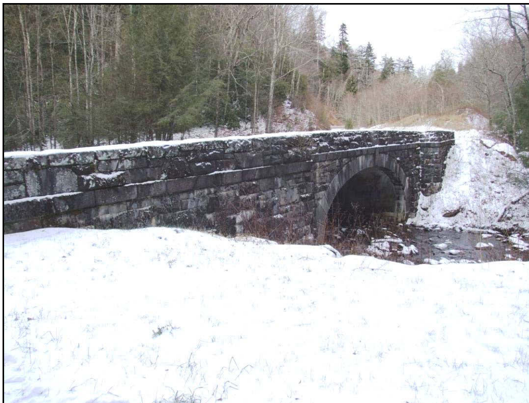
Figure 21. West Prong Little Pigeon Bridge.
