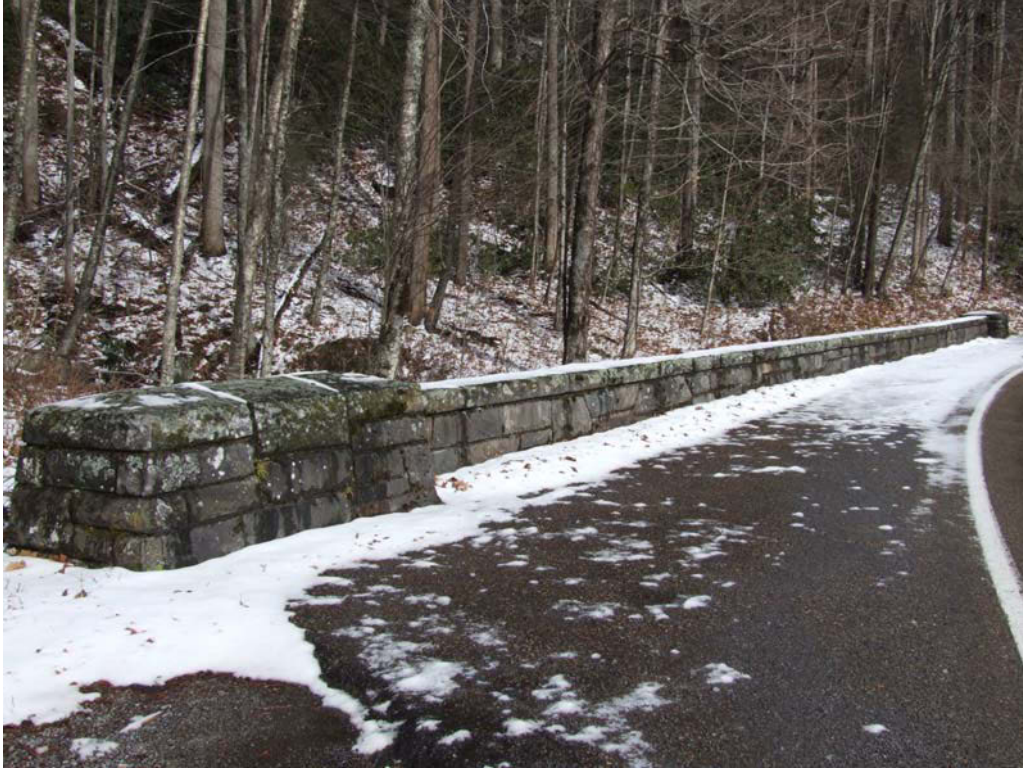
Figure 23. Cole Creek Bridge, Parapet and Pier.
