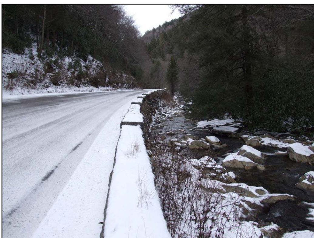
Figure 38. Crenellated Guard Wall/Retaining Wall, Milepost 11 (No. 188).
