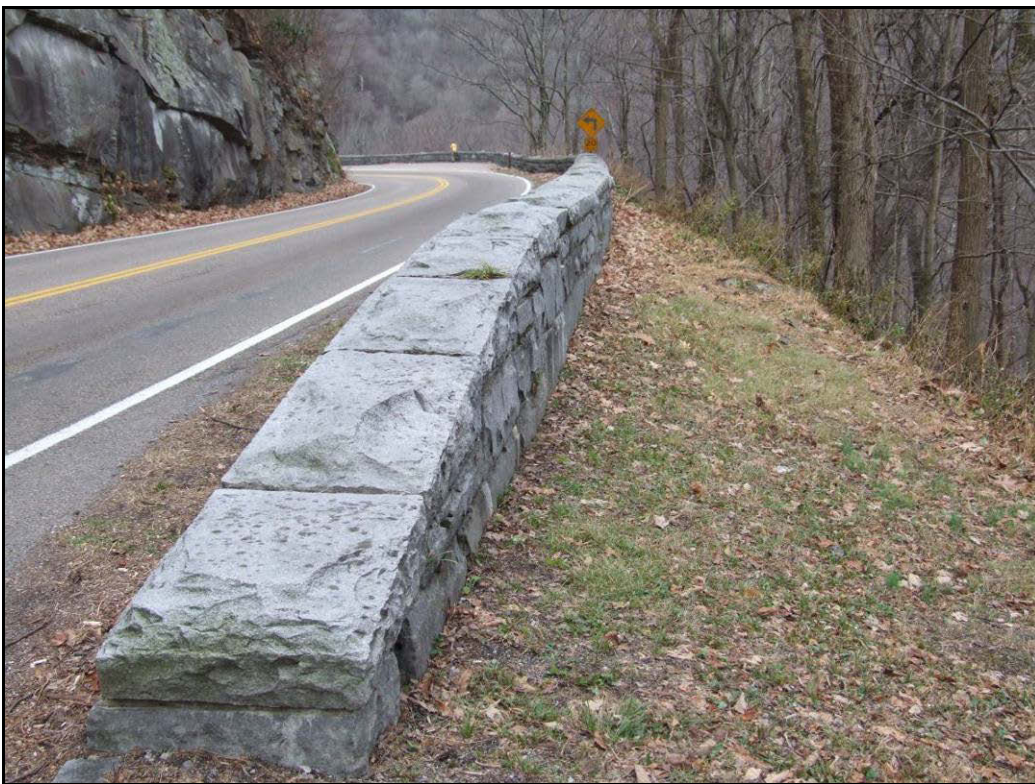
Figure 40. New Guard Wall Near Chimneys Trailhead, Milepost 7 (No. 103).
