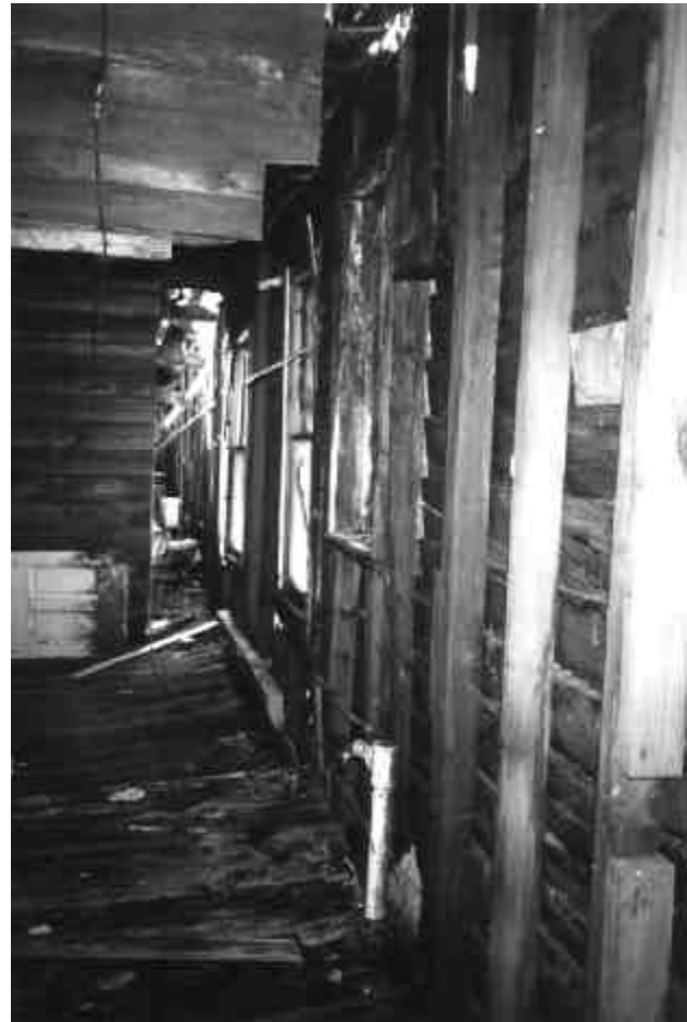
Figure 6.178. Wonderland Hotel, main section, second floor south wall, view east.
