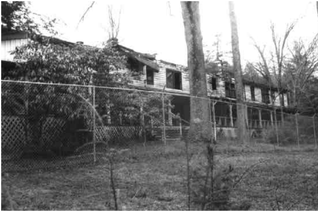
Figure 6.173. Wonderland Hotel, view of south side of main section.
