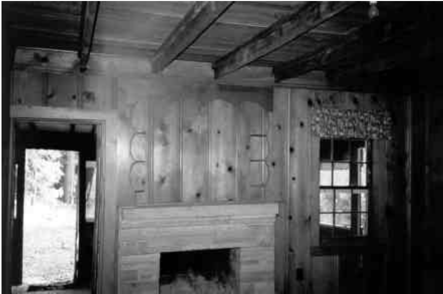
Figure 6.78. Andrews-Sherling Cabin (No. 21), interior view.
