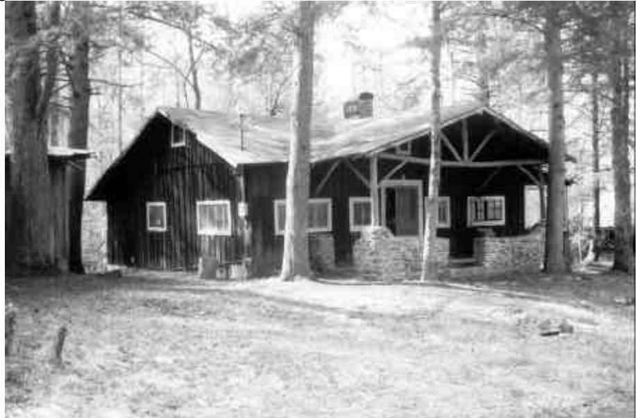
Figure 6.79. Congleton-Brownlow Cabin (No. 22), view of south & east sides.
