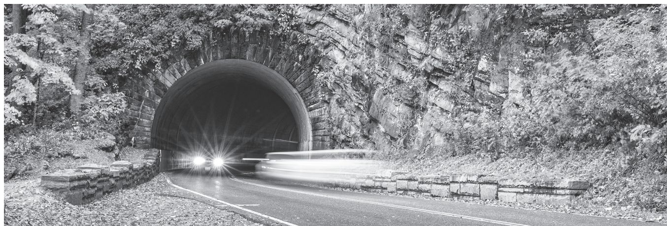
Roads, tunnels, and bridges within the park will benefit from Great American Outdoors Act funding. Image by Bill Lea.
