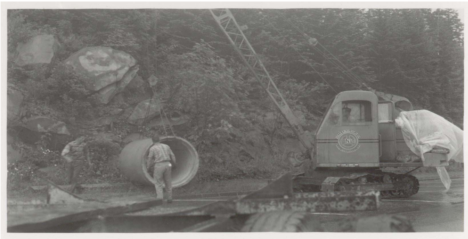
Fig. 7 "Loading Sections of Main Column at Clingmans Dome" NPS photograph by R.A. Wilhelm, 1959. Archives of GRSM.
