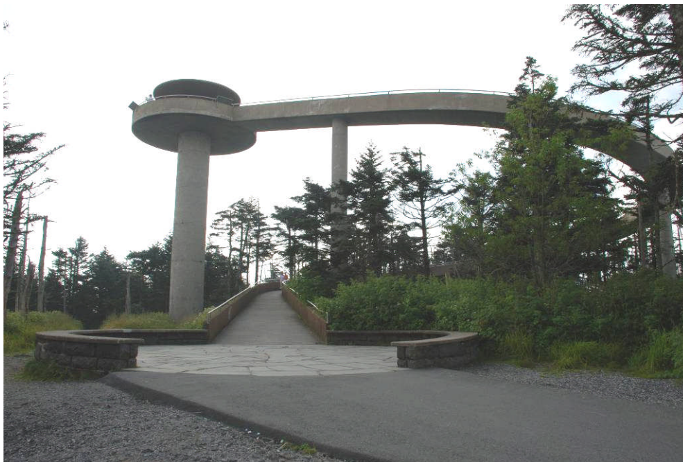
View to southeast, landing, ramp and observation platform
