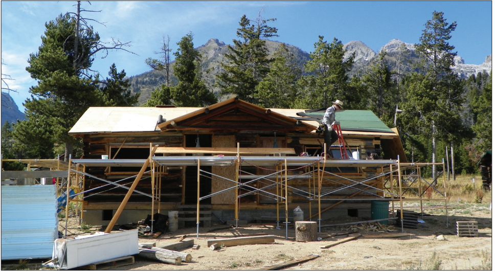
White Grass Dude Ranch Cabin undergoing rehabilitation work in 2008.
