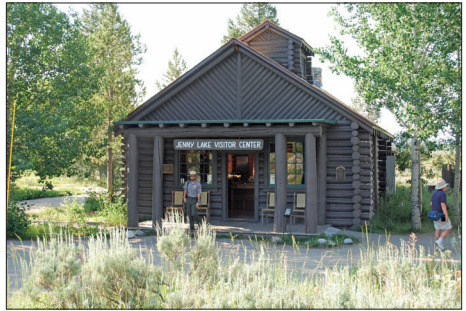
The Crandall Studio now serves as the Jenny Lake Visitor Center.
