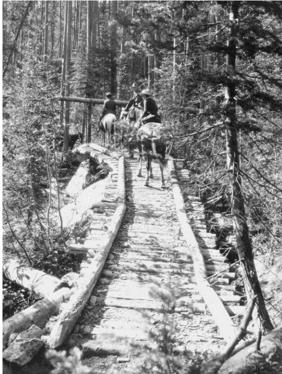
Figure 10. Trail building also meant facilitating passage across rivers and over wet places. CCC trail crews took pride in constructing bridges and other rustic crossings. By the time of MISSION 66, many of these features needed rebuilding.
