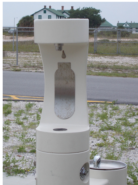
Water bottle filling station
