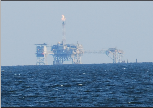
Offshore gas well south of Dauphin Island, Alabama.
