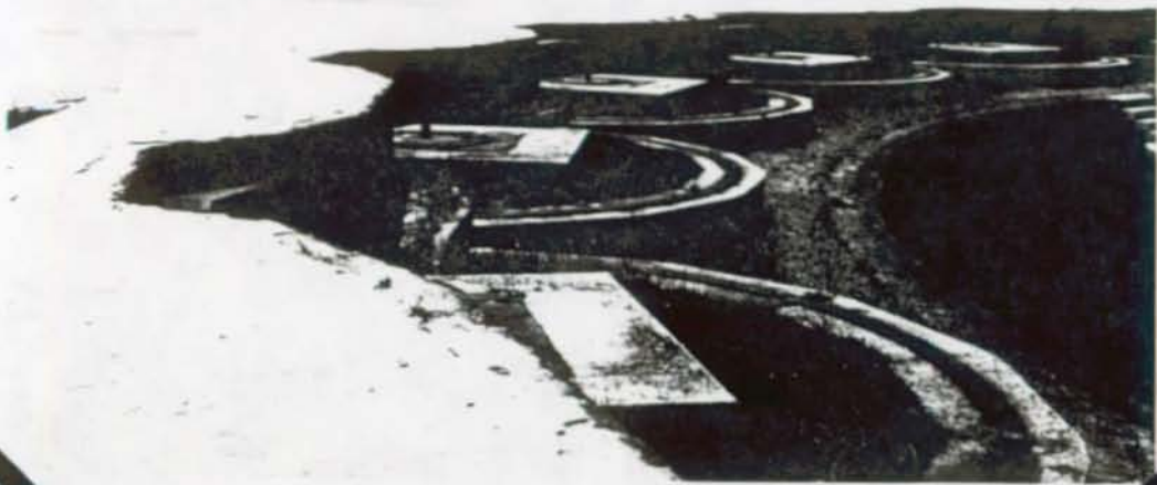
#3. View on top of parapet showing a few of the 21 gun mounts on upper rampart of Fort Massachusetts.
