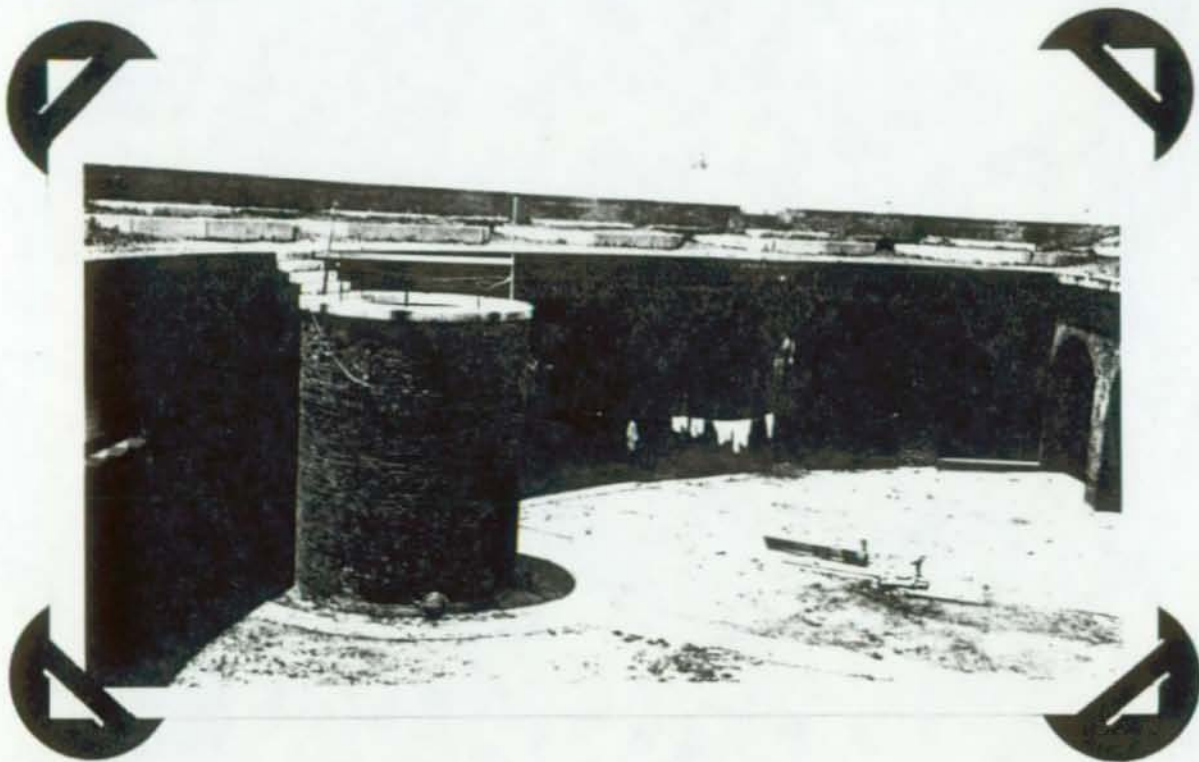
#5. An interior view of the Fort, showing one of the three circular brick stair-wells leading to the upper rampart. The laundry, screen doors and electric wiring are all modern innovations.
