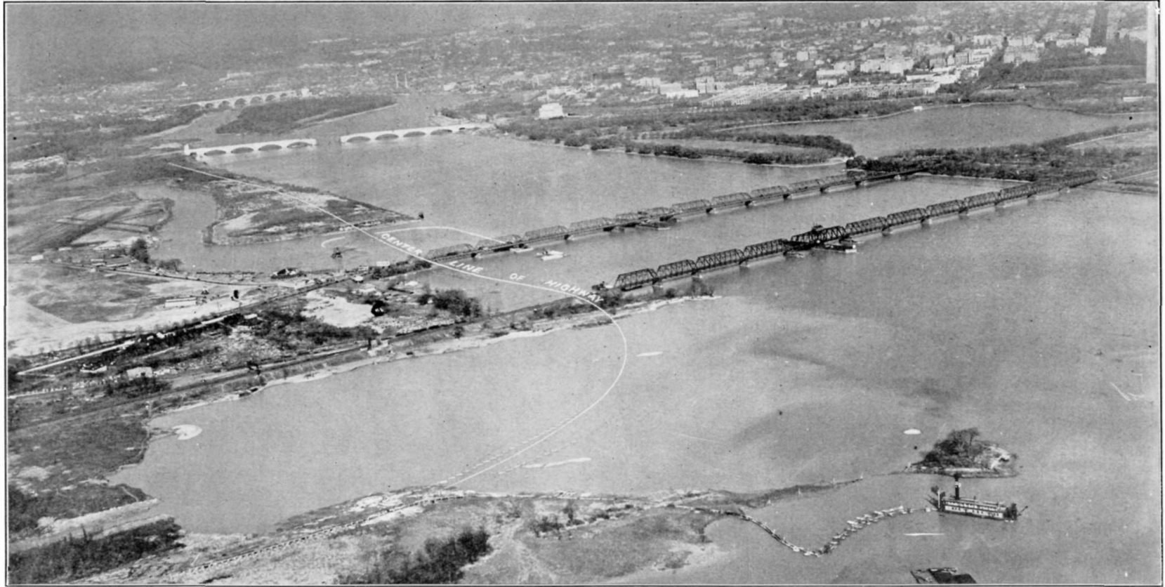
FIGURE 4.—Airplane view of the area which will be occupied by a highway grade separation structure and connecting ramps at the south end of the Highway Bridge across the Potomac River, taken during the first stages of placing hydraulic fill. The riprap foundation for seawall to inclose the river side of the fill to be placed at this location appears as a white line. The plans provide for the removal of the two southerly spans of the Highway Bridge and the replacement of the roadway on earth fill, which will permit direct access to the Highway Bridge from the Memorial Highway over a connecting ramp
