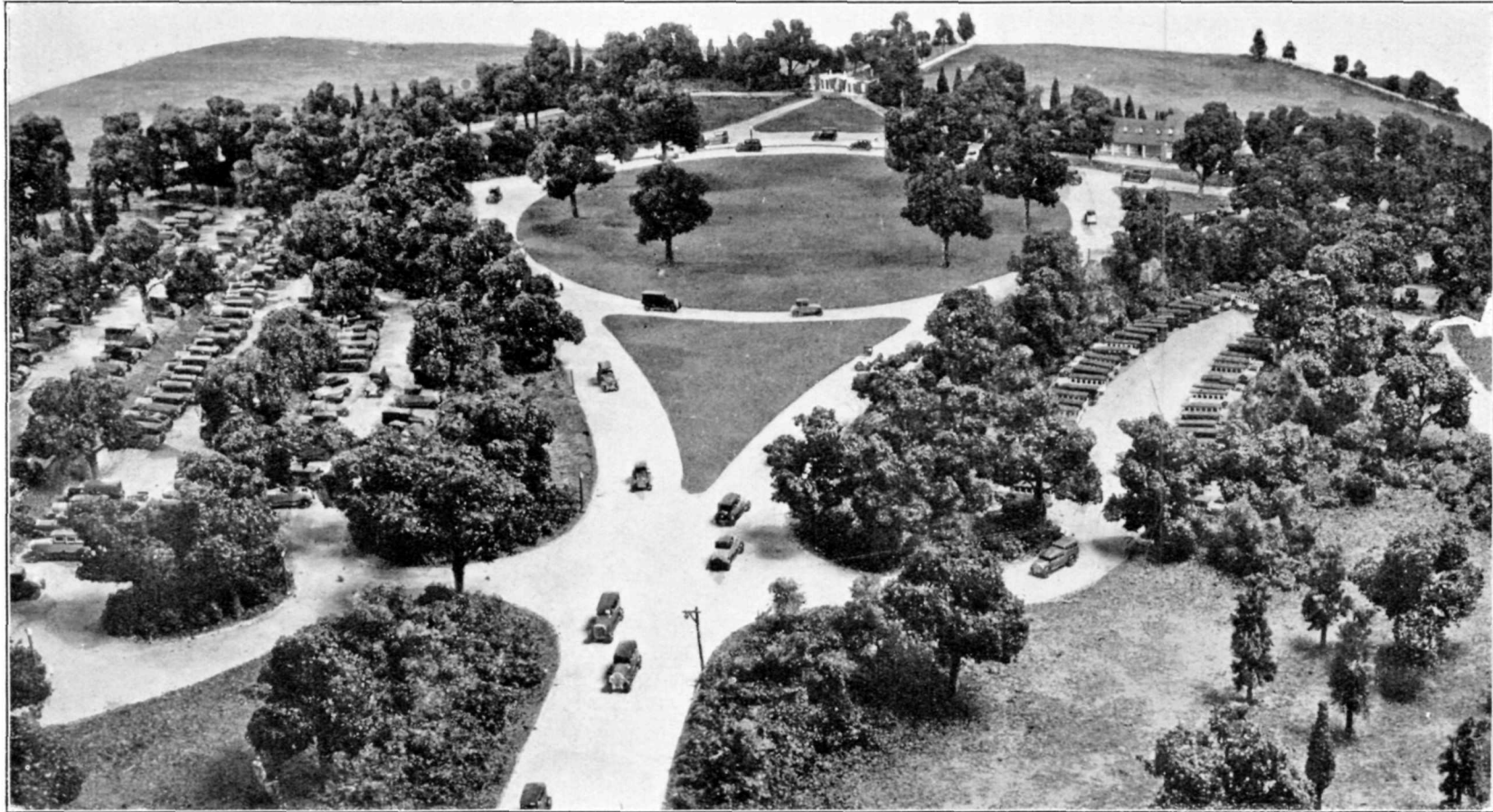
FIGURE 17.—Photograph of a model, constructed to scale, of the Mount Vernon terminus of the project as planned, showing the provision for traffic circulation, parking, etc.
