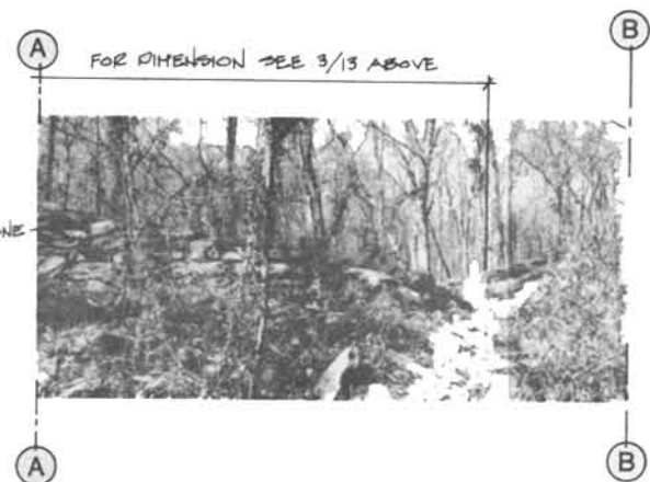
4 13 SOUTH END OF HOLDING BASIN WALL / LOOKING WEST FROM OUTSIDE OF BASIN
