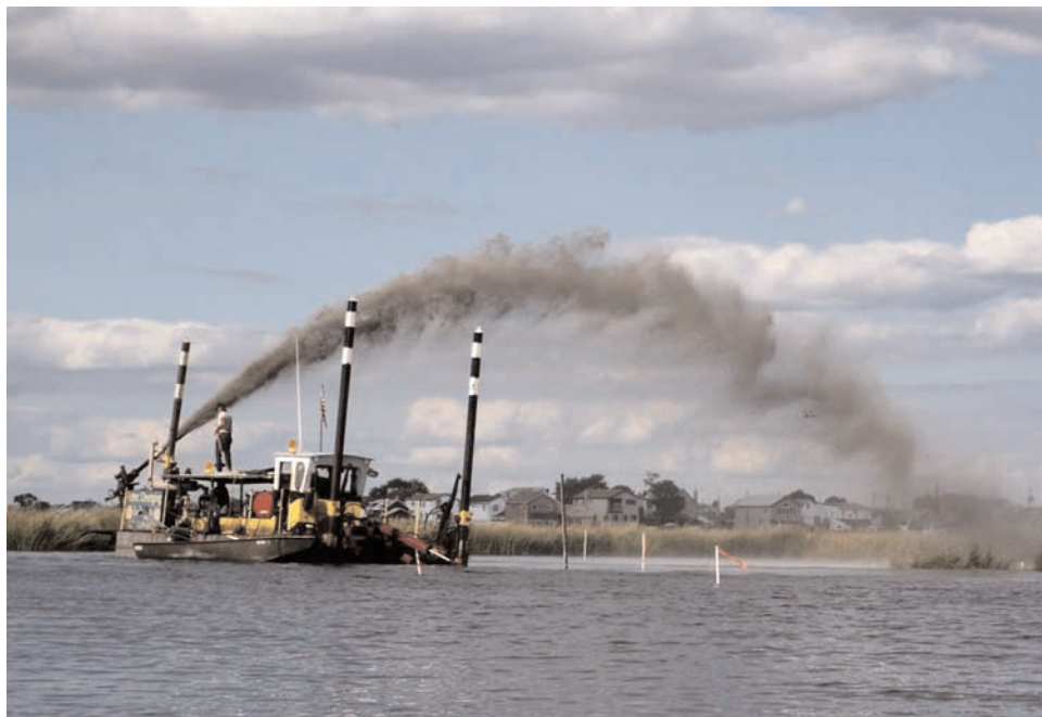
Figure 1. A swing-ladder dredge with high-pressure spray extracted 6,000 cu 3 of sand from a trench in the adjacent creek and sprayed it over the surface of Big Egg Marsh.
