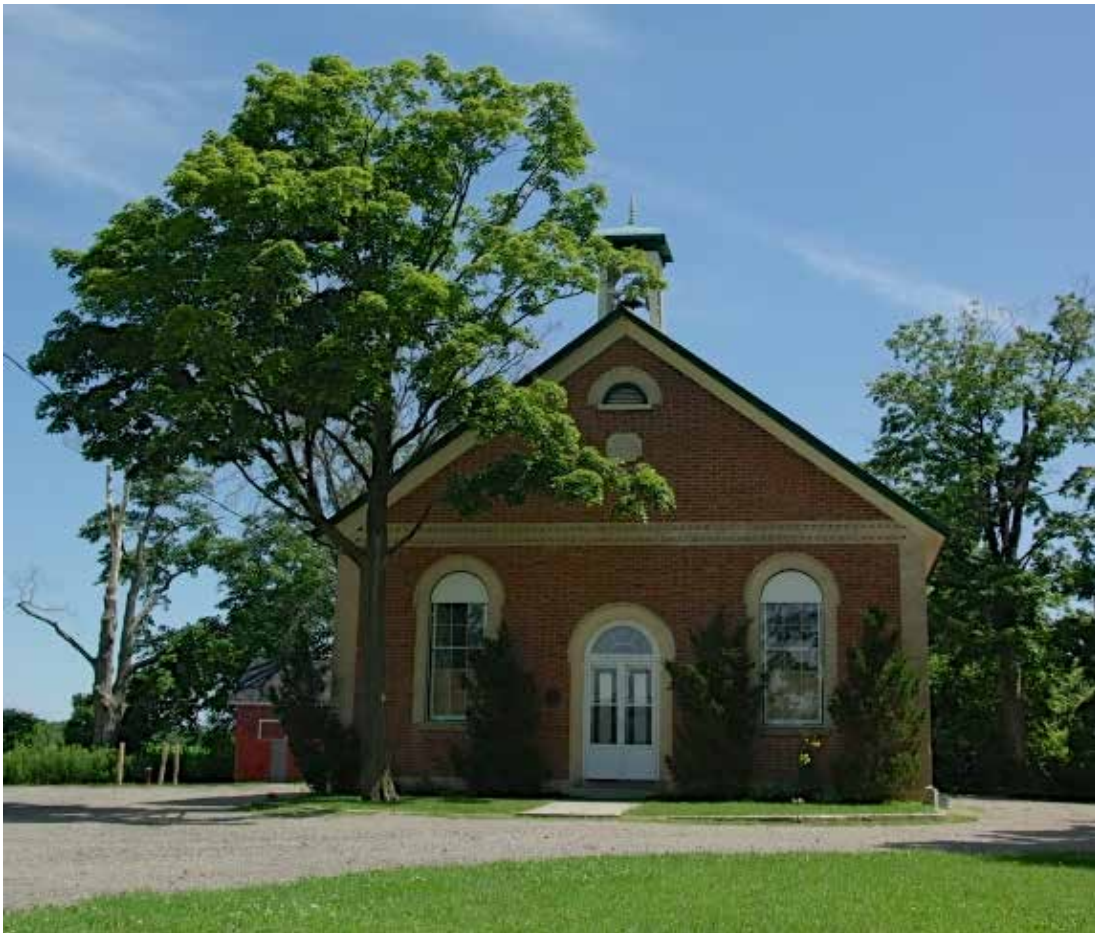
Figure 1. Rouge Park has many historic structures. Photo courtesy of Rouge Park.
