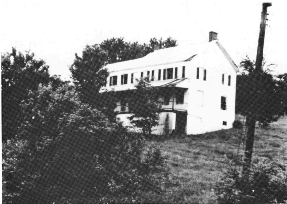
Otto House at the Antietam National Battlefield in Sharpsburg, Maryland. Photographer: Joseph D. Balachowski, 1988
