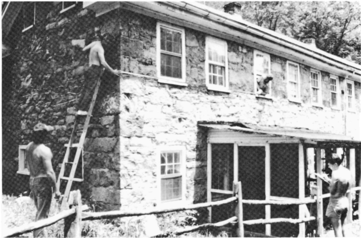
Bill Richardson, owner of the Mt. Etna Barracks in Etna, Pennsylvania, watches team members Mark Pierson, David Kalhoefer, and Gilbert Witte measure the structure. Photographer: K. Edward Lay, 1988
