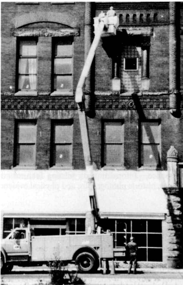
Left, using a cherry picker to photogrammetrically record the Masonic Temple. Right, close-up view showing Anette Jensen measuring a window, with the assistance of a cherry picker. Photographer: K. Edward Lay
