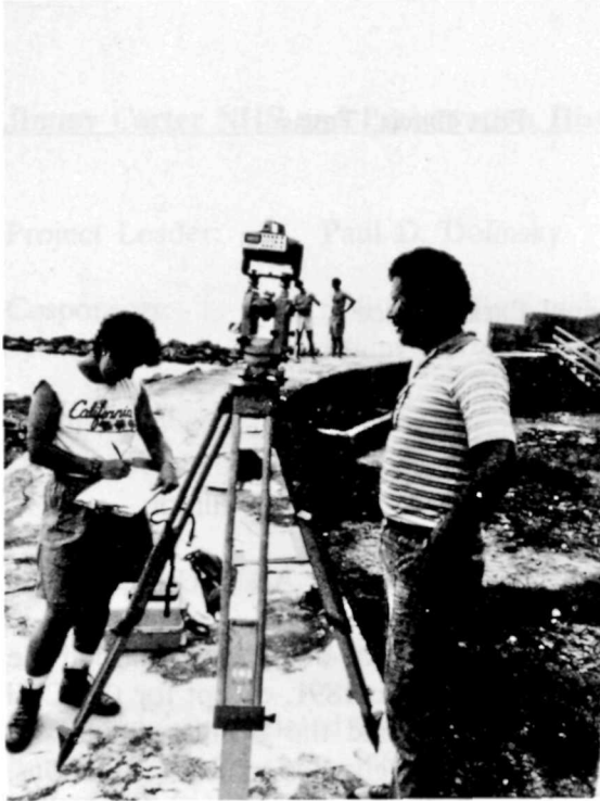
EL MORRO. Jacqueline Salame (l) jots down readings translated by Erick Chaves (r) from the theodolite. Background , Matt Wiencek (l) and Chris Huckabee (r) work with target.
