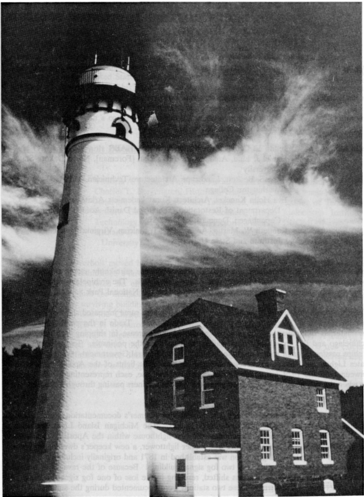
Outer Island Lighthouse Apostles Island National Lakeshore Bayfield, Wisconsin Photographer: Kenneth W. Martin
