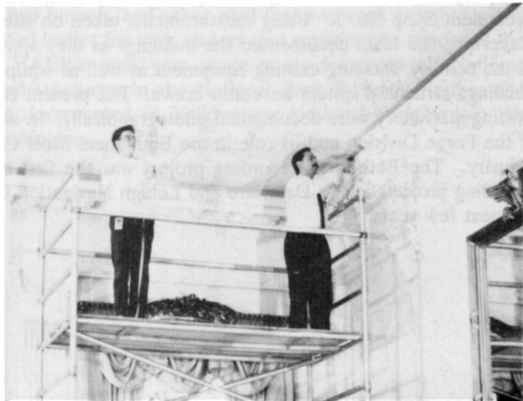
Douglas Anderson (left) and Robert Arzola (right) measure the ceiling of the East Room at The White House. Photographer: Frederick Lindstrom
