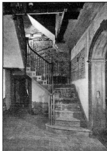
Stair Hall under restoration, Belair Mansion, Bowie, Prince George's County, Maryland (HABS No. MD-87-43). Photographer: Jack E. Boucher - 1994.
