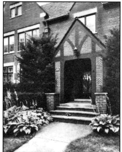
Entryway, Wright-Patterson Air Force Base, Brick Officers' Quarters, Types C & D, Dayton vicinity, Green County, Ohio (HAER No. OH-103-C). Photographer: Dave Diesing, Hardlines - 1994.
