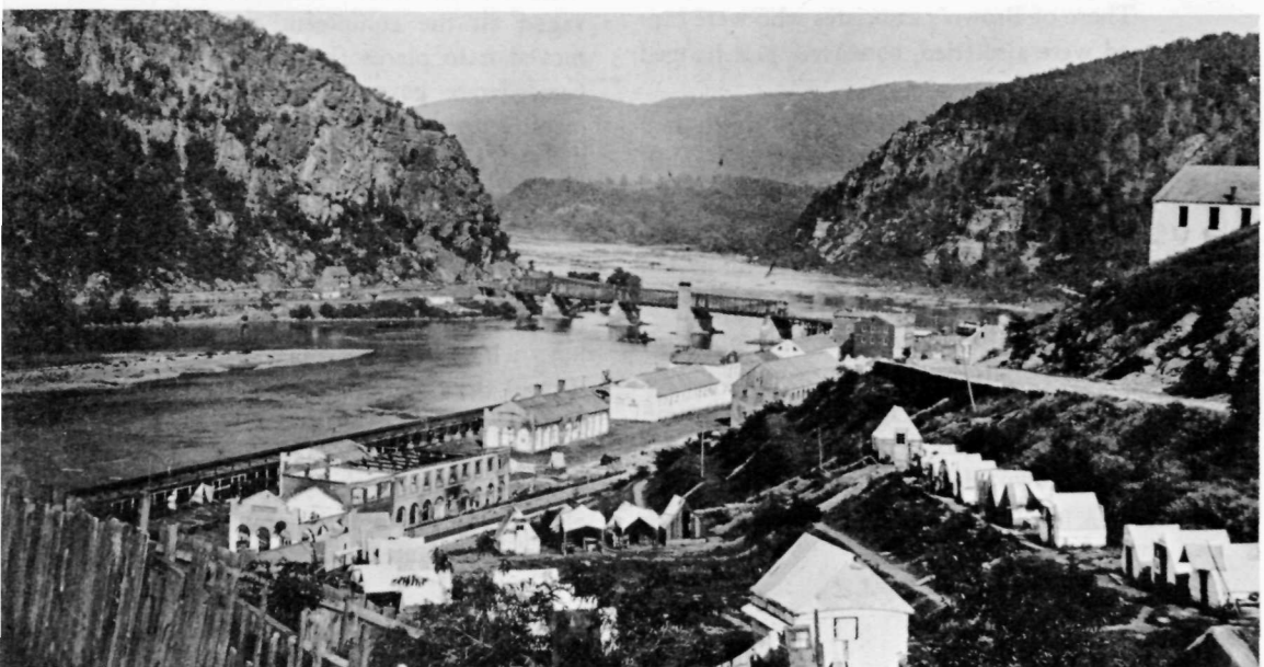
Harpers Ferry, near the end of the war. Ruined armory buildings on the left. Courtesy, Library of Congress.
