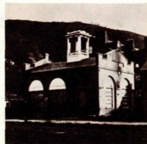
The fire enginehouse
