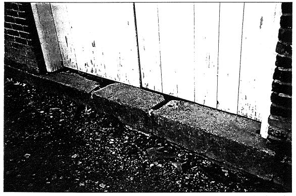
Figure 5 - John Brown's Fort , dressed stone water table at north elevation. Note deteriorated mortar joints.
