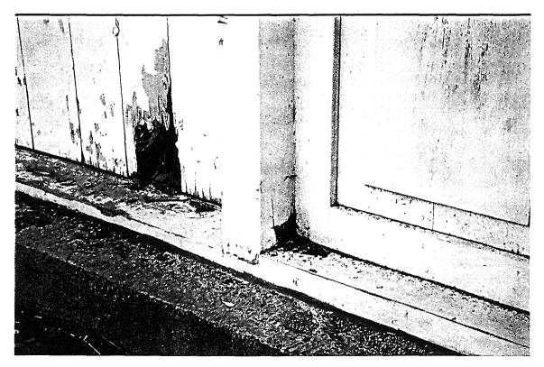
Figure 10 - John Brown's Fort , detail at bottom of door and sidelight showing rot.
