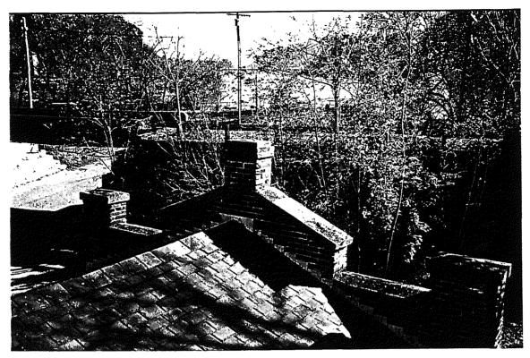
Figure 13 - John Brown's Fort, interior of east end wall above roof. Note stone caps and lack of mortar wash on chimney features.
