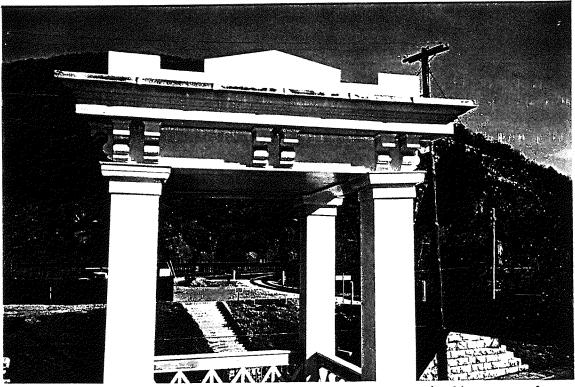
Figure 17 - John Brown's Fort, south elevation of cupola. Note top of column capital at front right slopes inward.
