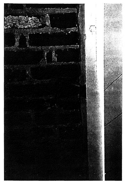
Figure 12 - John Brown's Fort , interior elevation of jamb at center bay doors. Note wood nailing block pulling away from masonry.
