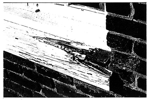
Figure 8 - John Brown's Fort, rot at window sill of northern most window at east elevation.
