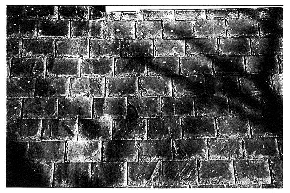
Figure 16 - John Brown's Fort, plan view of slate roof with one broken slate shown in center. Note trim at base of cupola is tight to slate.
