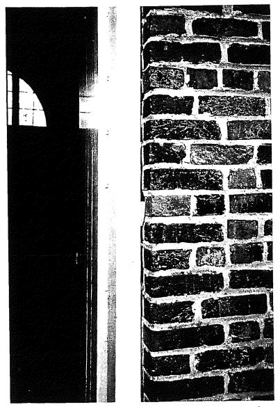
Figure 11 - John Brown's Fort, wood jamb of double doors at center bay. Note gap between wood and masonry.
