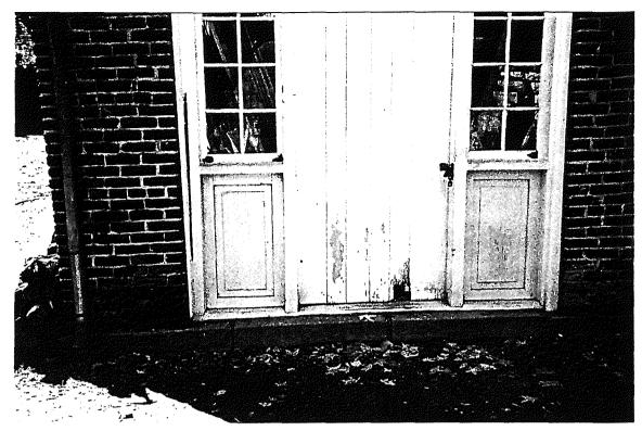
Figure 9 - John Brown's Fort, door and sidelights at eastern bay of north elevation. Note gutter discharges at base of building.
