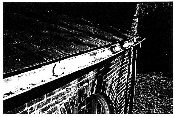
Figure 19 - John Brown's Fort , half round gutter on south elevation. Note how shape has flattened out and is wavy.
