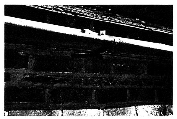
Figure 20 - John Brown's Fort , detail of gutter hanger and strap.
