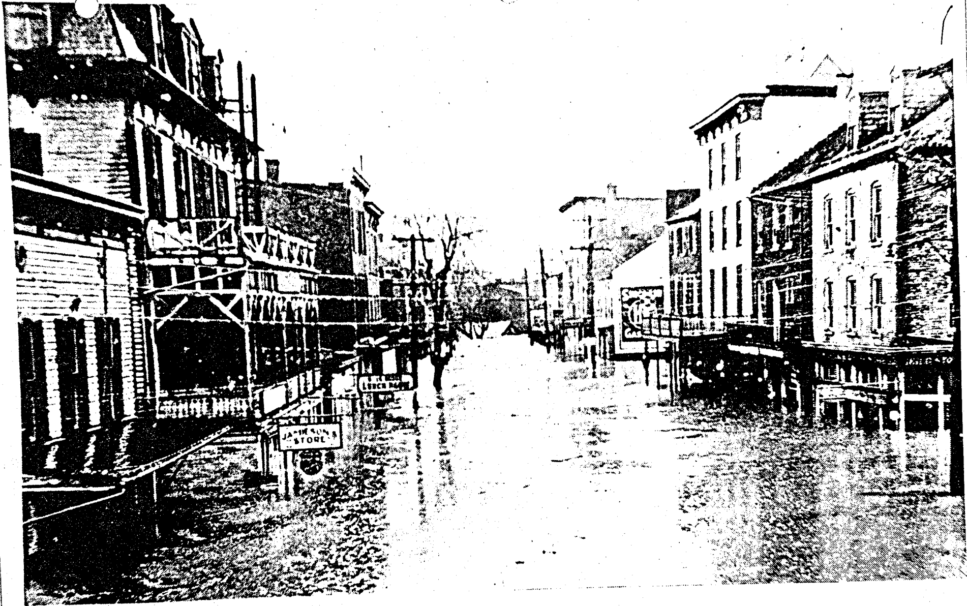
HF- 281 Harpers Ferry in 1936 Flood. Bldg. No. Three story structure in distance at far right center.
