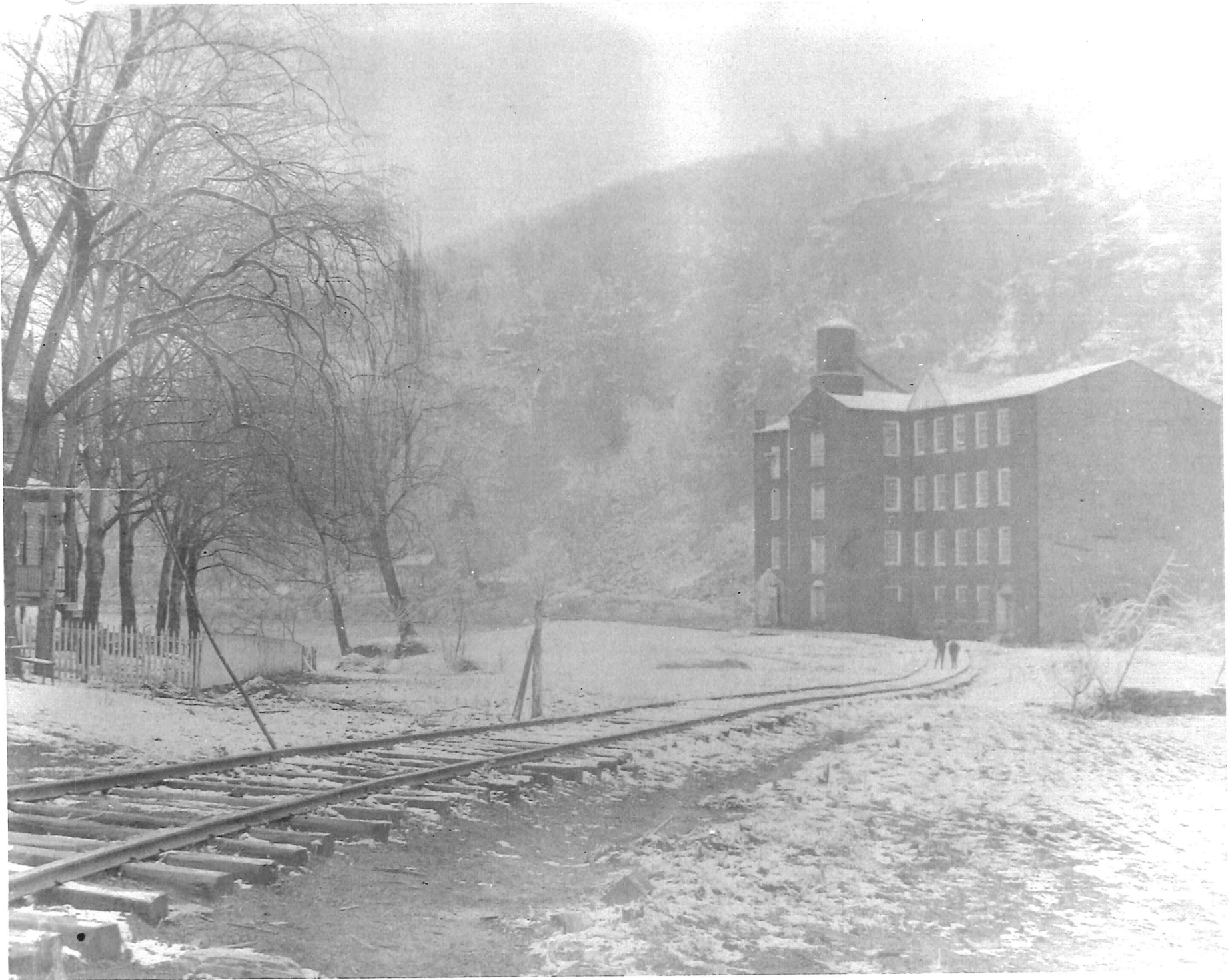
Photograph 9. HF-897, Virginian Island, showing 2-story frame structure at left, probably taken after 1902.
