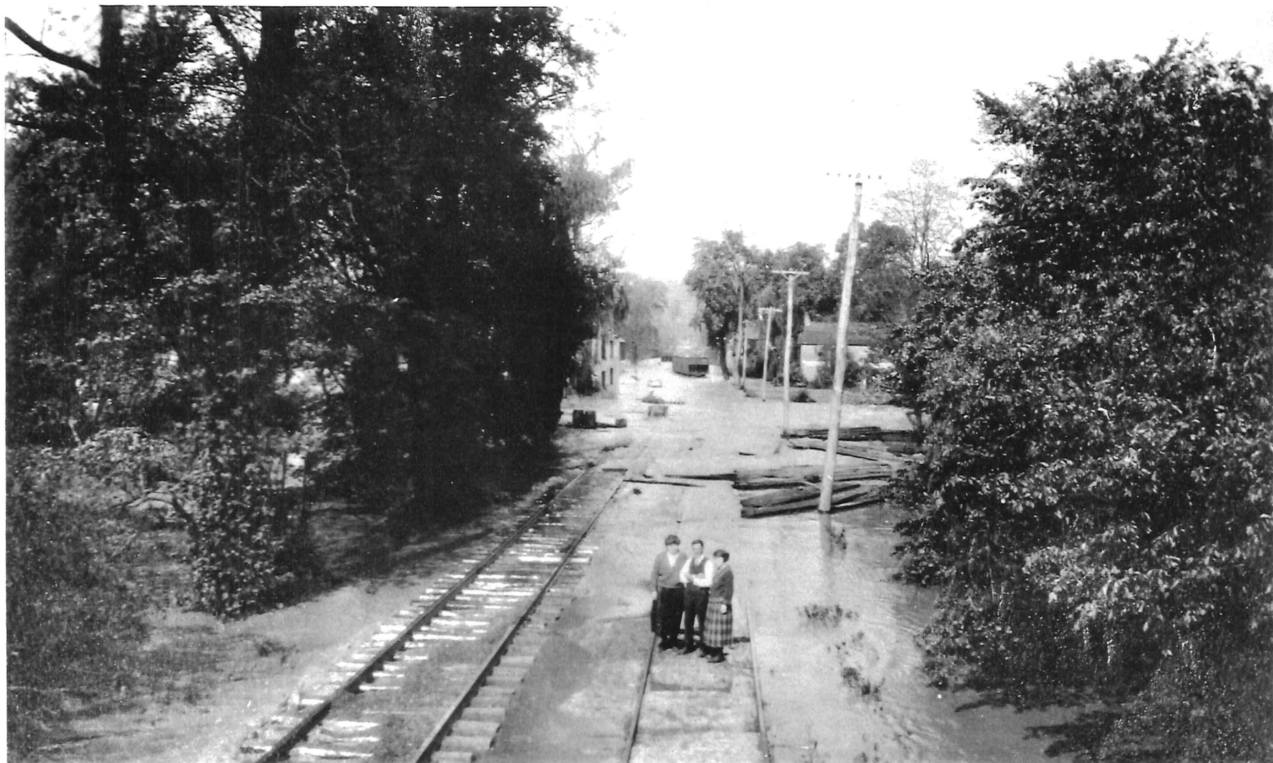
Photograph 12. HF-1311, View along the tracks looking west during 1924 flood.
