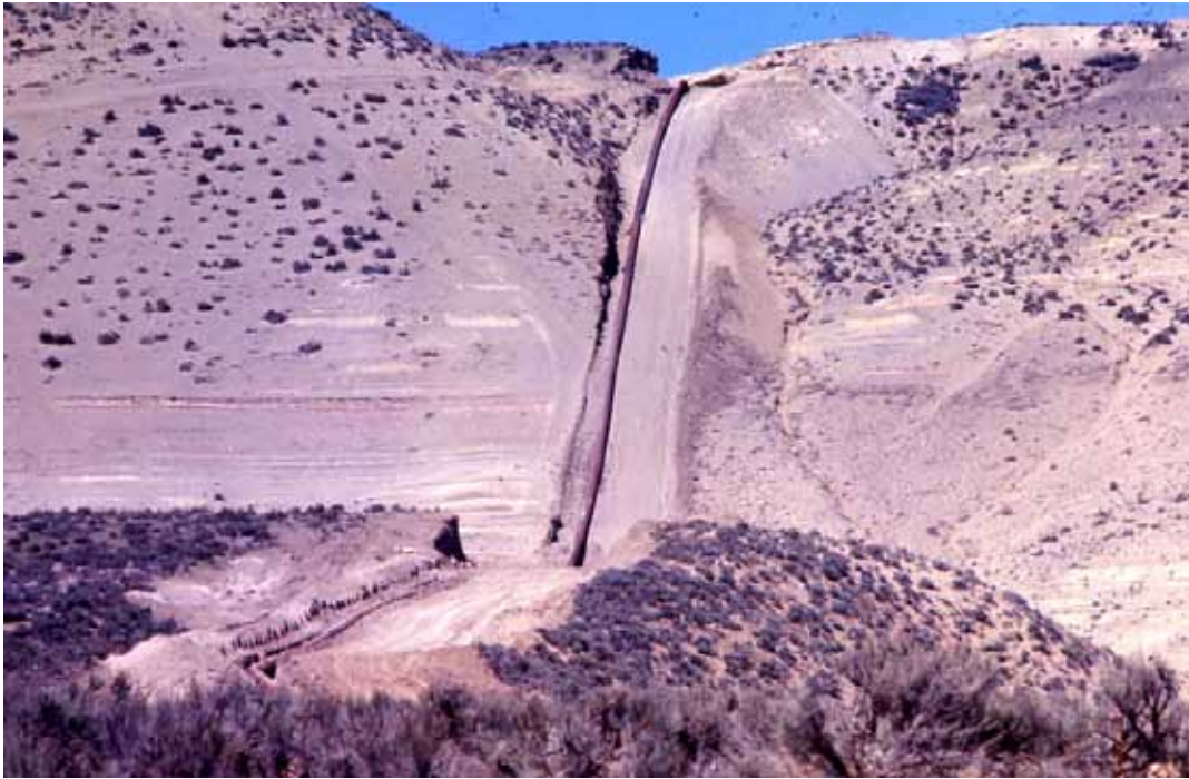
Figure 12. Construction of pipeline transporting water from the Snake River to the Bruneau Plateau. The completed pipeline includes three pipes. The trench is now filled in. Interestingly, the vegetation on the slopes results from seepage of groundwater from irrigation activities. Naturally the slopes are unvegetated. NPS photo courtesy Phil Gensler (NPS HAFO).
