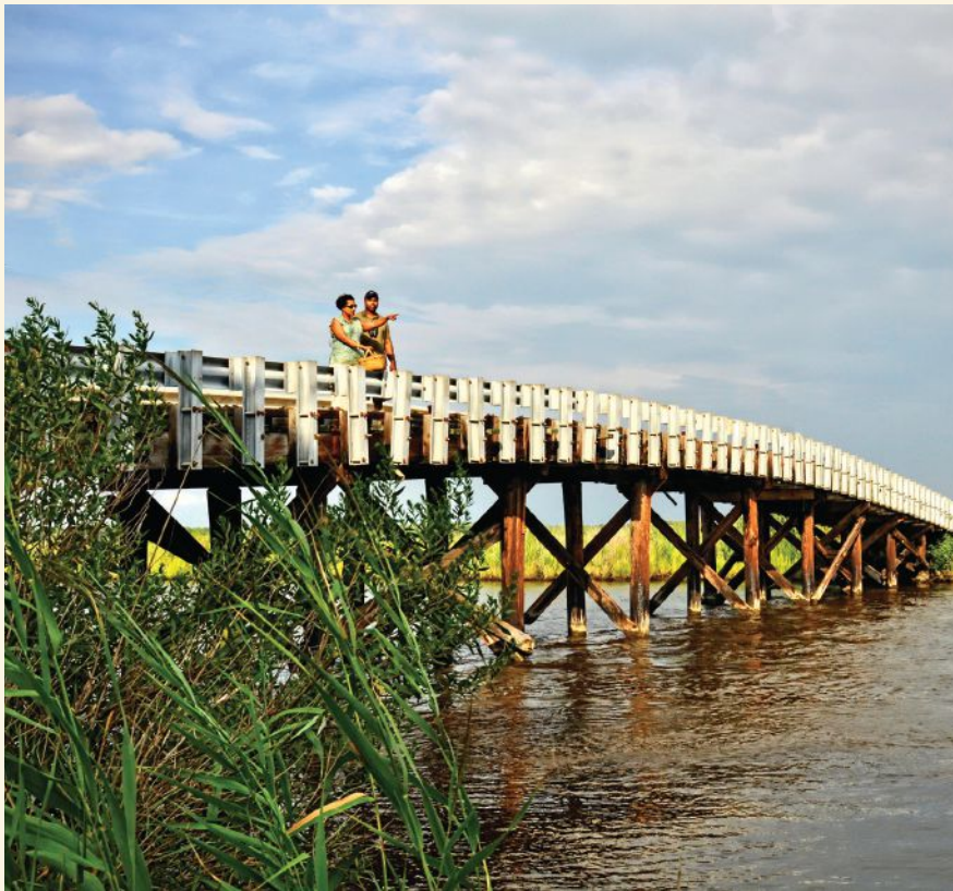
Bestpitch Ferry Bridge, a one-lane wooden bridge, is located at the site of a former ferry over the Transquaking River.
