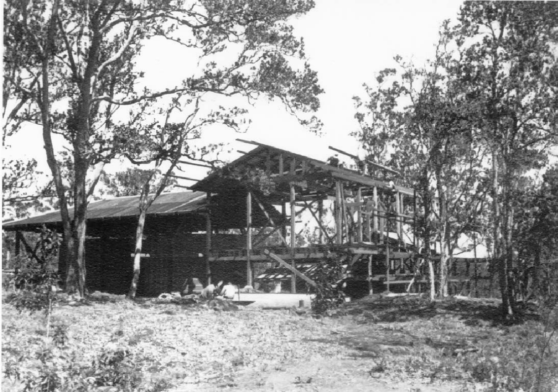
Physical History # 1: Historical photo of the construction of the 'Ainahou Ranch House (courtesy of Samuel M. Lowrey, 1941).
