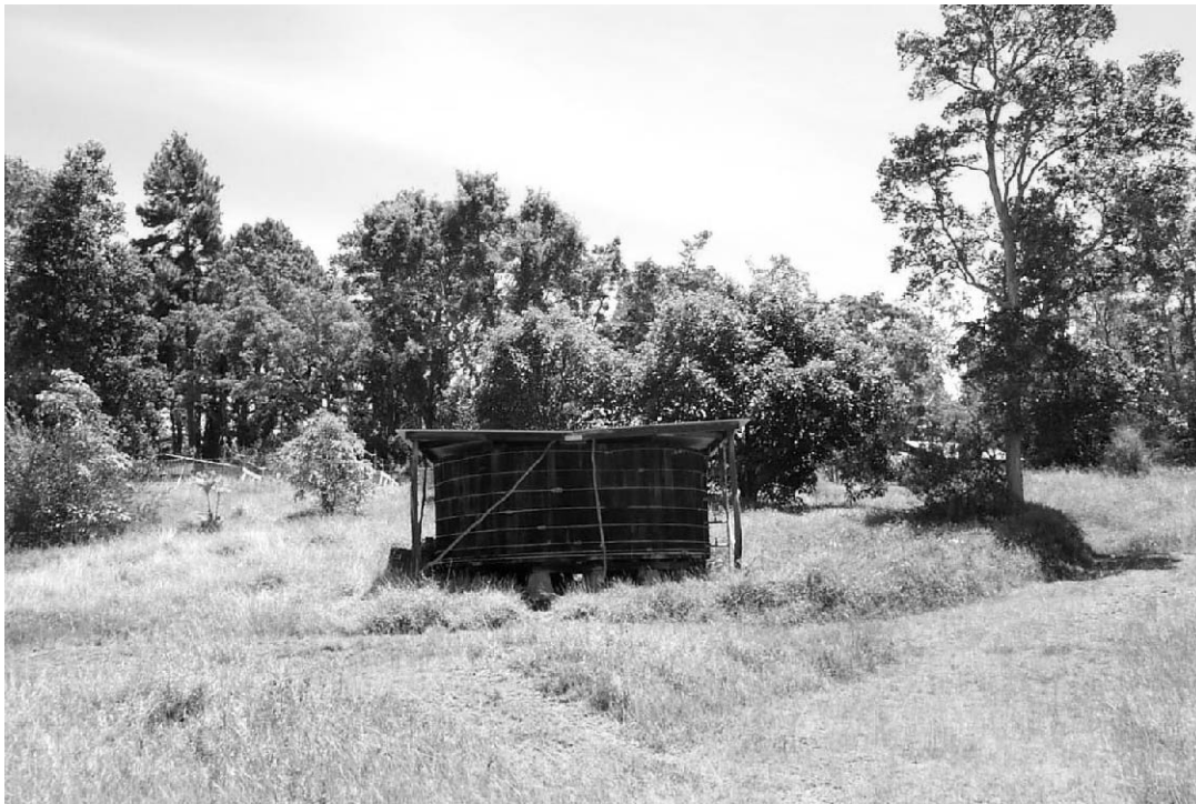
Topography # 1: In Shipman's gravity-powered water system, this water tank a few feet down from the nursery area collected water from the roofs of the hothouses, and serviced the livestock facilities down slope (PWR, HAVO, CLI files, 2003).
