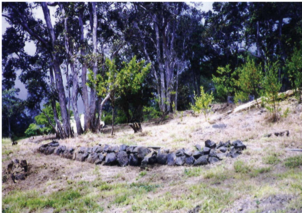
Buildings and Structures # 6: A dry-laid lava rock retaining wall located between the nursery area and the ranch house (PWR, HAVO, CLI files, 2003).
