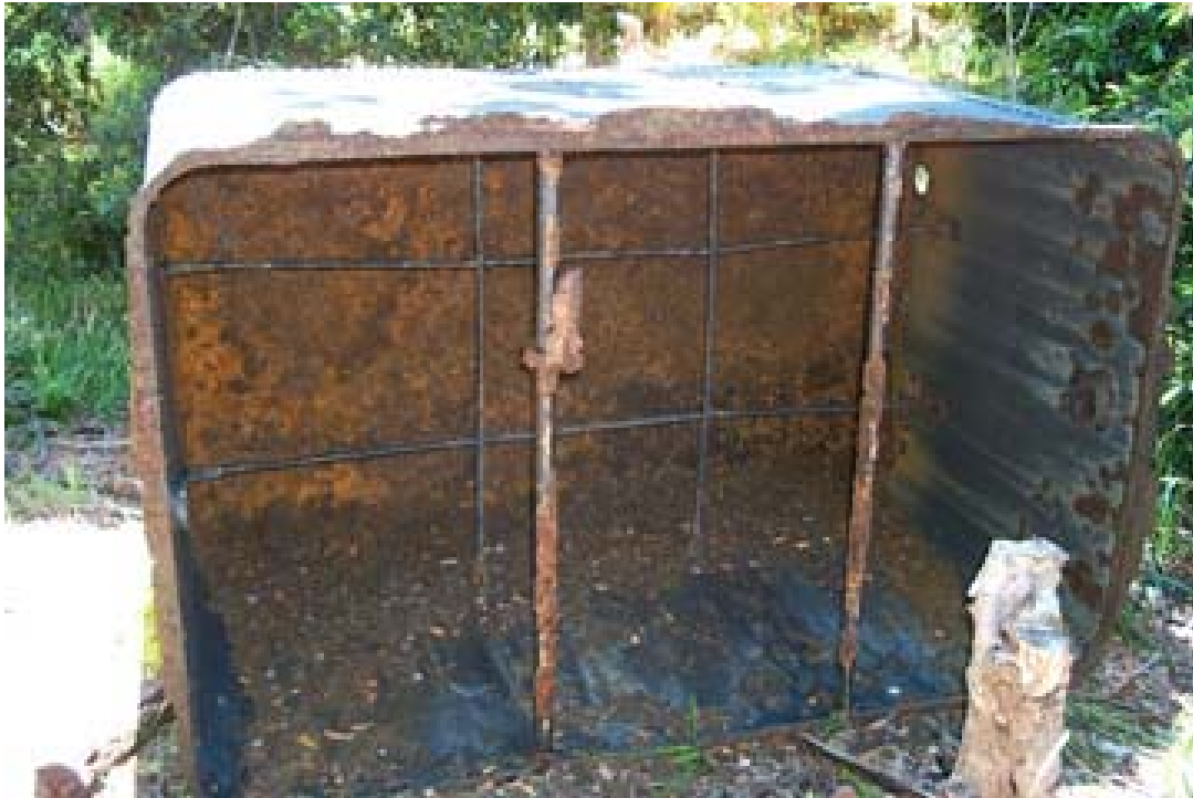
Buildings and Structures # 7: A rusty metal container near the generator shed foundation. Historical function unknown (PWR, HAVO, CLI files, 2003).
