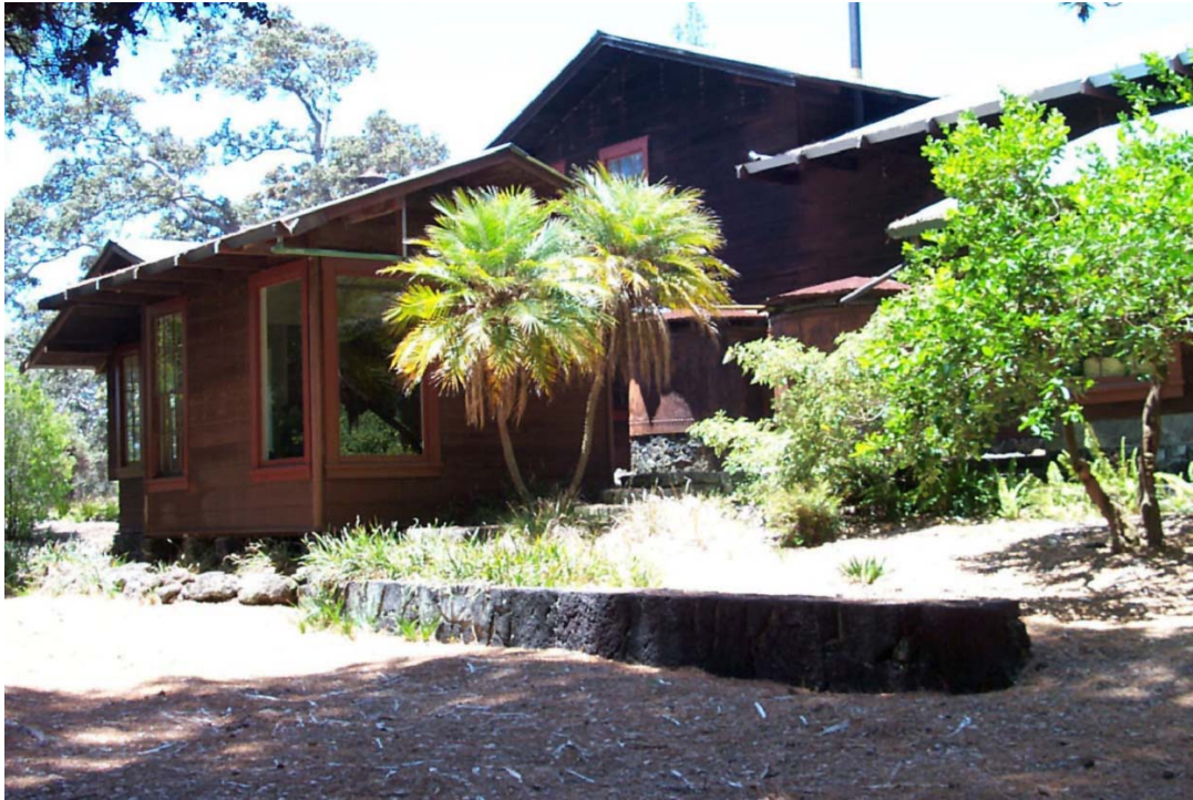
Buildings and Structures # 3: Contemporary photo of the east side of the ranch house (looking SW)(PWR, HAVO, CLI files, 2003).
