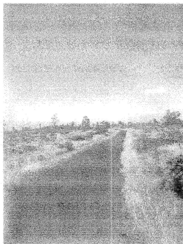
Toward the end of Hilina Pali Road, the vegetation becomes predominantly grassland, and the road descends and winds with average grades of 5% until the end of the road.
