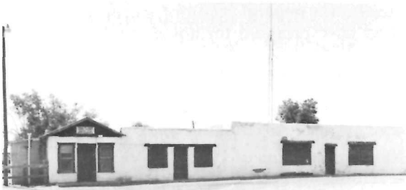
Former Housing Authority Building.
