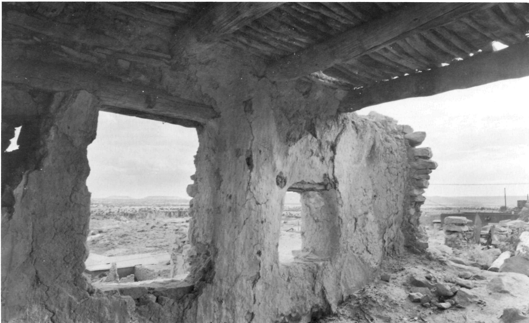
Latias were placed on top of the vigas in a perpendicular pattern. Latias are thin branches, usually 1.5–4 inches in diameter, which were topped by another layer of willows, yucca, or saltbrush, and then covered with a layer of mud.
