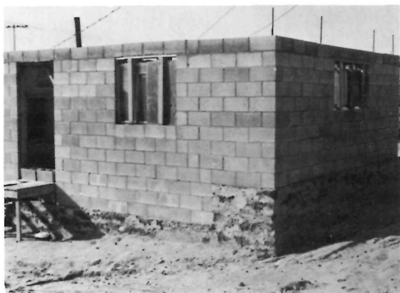
Structures of cement block construction covered with cement stucco can be made to look like traditional stone and adobe houses. As in other new housing units, these block houses feature modern doors, windows, and interior details.
