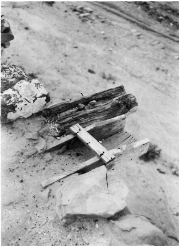
Drainage from a flat roof can be a problem. Some early houses were built so that the vigas and the entire roof line sloped, directing the drainage water down to the canales, or drainpipes. Before sawn lumber and sheet metal became available, canales were made of stone or hollowed logs.
