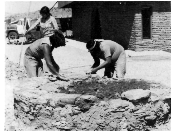
The Arts and Crafts Center encourages Lagunas to learn traditional skills and technology of masonry building, like the bread oven construction pictured above.
