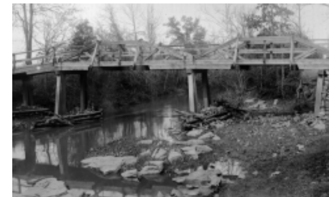
Reed’s Bridge, located near the site of the first battle of Chickamauga, was originally a three-span timber truss. This bridge has been replaced twice. (CHCH)
