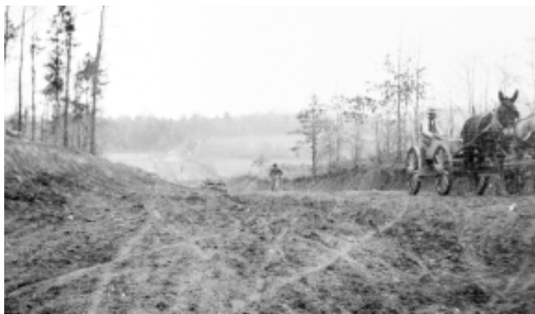
Roadwork included improvements on approach roads to the park, such as Ringold Road, ca. 1893. (CHCH)
