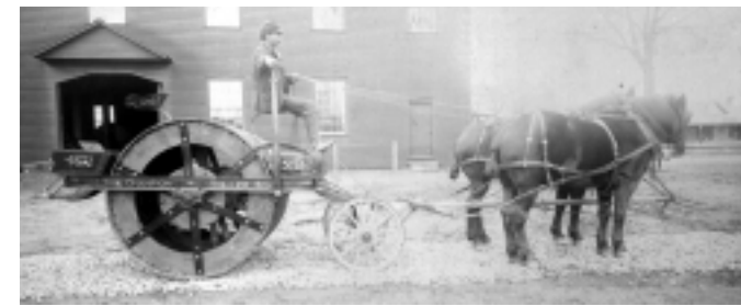
Horse-drawn equipment and hand tools were used to construct park roads, ca. 1893. (CHCH)
