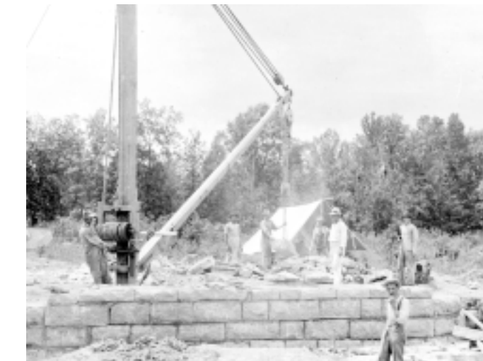
Hand labor was used for much of the construction work. Derricks placed large stones for culverts and bridges. (CHCH)
