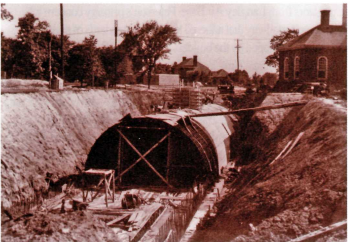
Tunnel under construction through the Courthouse Green, 1930s. (CW)
