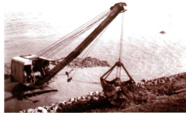
Laying of rip rap for seawall construction along the York River, 1935. (COLO)
