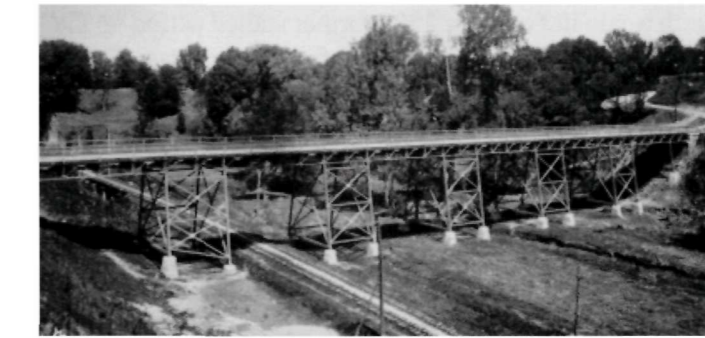
Stouts Bayou Bridge, ca. 1903, was replaced with a similar steel girder span in 1937. (VICK)
