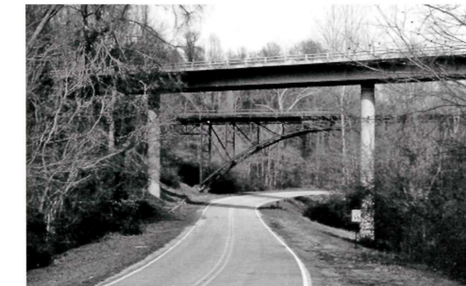
The Steel Bridge spanning Jackson Road was by-passed with a modern concrete span in 1972, but remains alongside. (HAER)
