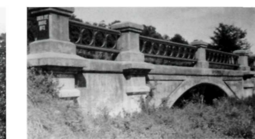
▲ Original wrought iron railing of the Melan-type bridges, ca. 1903. (VICK) ◀ View of Melan bridge along Union Avenue. (HAER) ▶ HAER drawing illustrates the varying sizes and shapes of arch spans (G.Seale)
