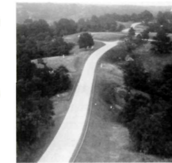
Before and after view of Confederate Avenue reconstruction by the CCC, ca. 1930s. (VICK)
