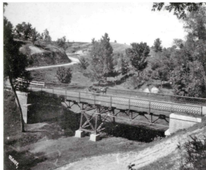
Steel viaduct spanning Glass Bayou on Union Avenue. Constructed ca. 1903, later destroyed during rerouting of the tour roads. (VICK)
