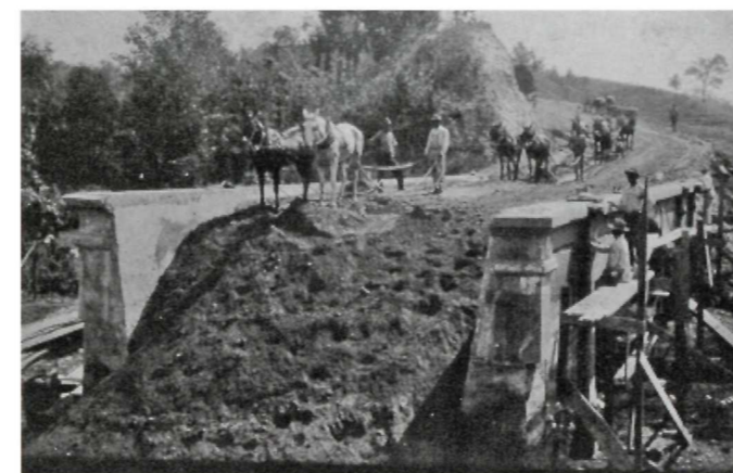
Roadway and Melan arch bridge under construction along Union Avenue, ca. 1903. Horse-drawn equipment was used to grade the roadbed. (VICK)
