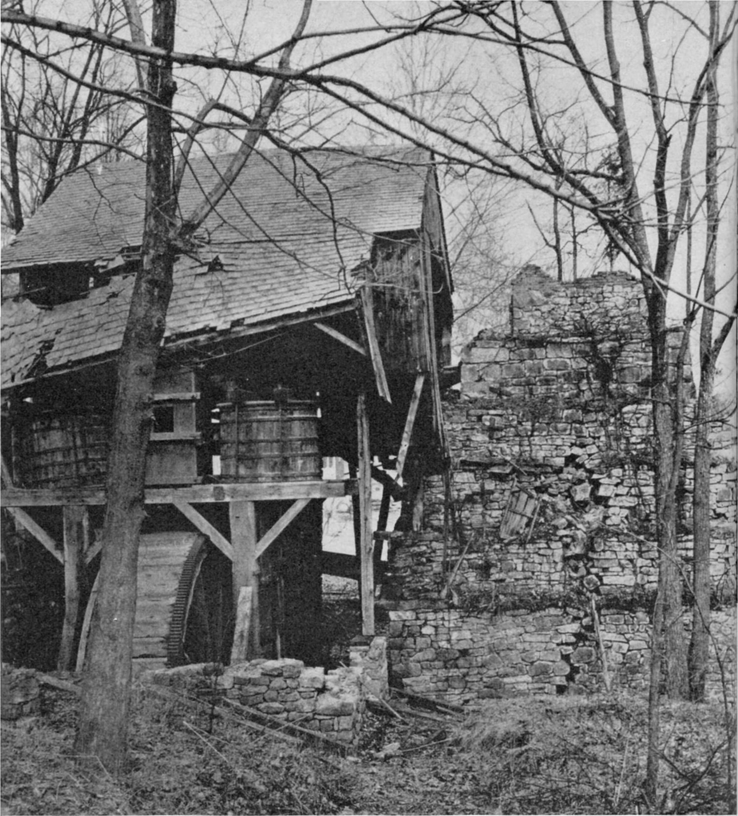
Hopewell Furnace and its blast machinery about 1925. The machinery is no longer in place, but its reconstruction is contemplated by the National Park Service as part of a general plan to rehabilitate Hopewell Village
