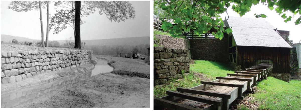
Figure 6. Water was needed to drive the water wheel powering the blast machinery. The east head race (left; 1939 photo after retaining wall restoration) and west head race and flume (right; 2006 photo after reconstruction) were man-made structures that transported water to the wheel house. Their locations are indicated on figure 1. National Park Service photographs in Yocum (2008).
