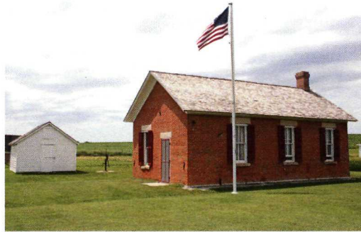
The Freeman School as it appears today. NPS photo
