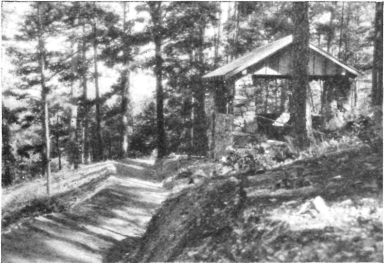
SHELTER HOUSE AND TRAIL ABOVE IRON SPRINGS, HOT SPRINGS MOUNTAIN
