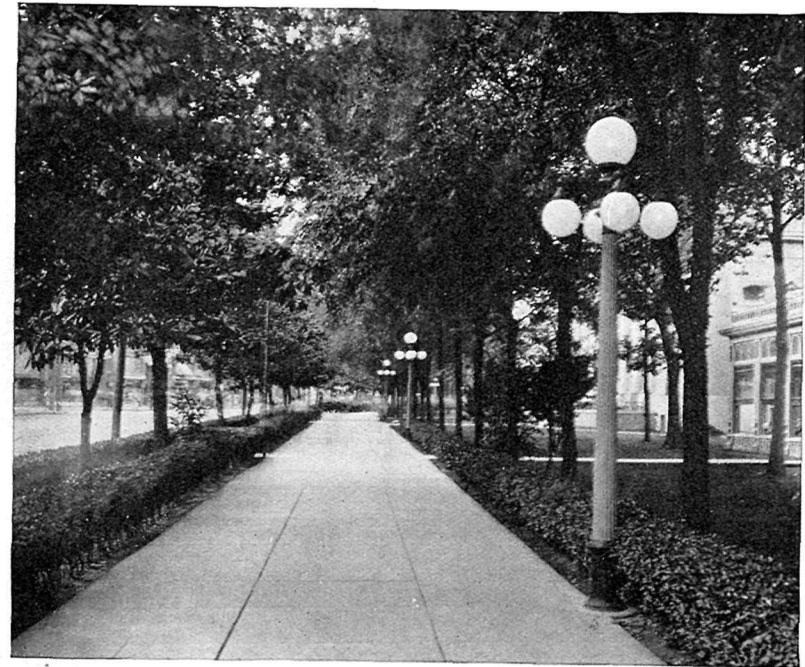
MAGNOLIA PROMENADE ALONG BATHHOUSE ROW
