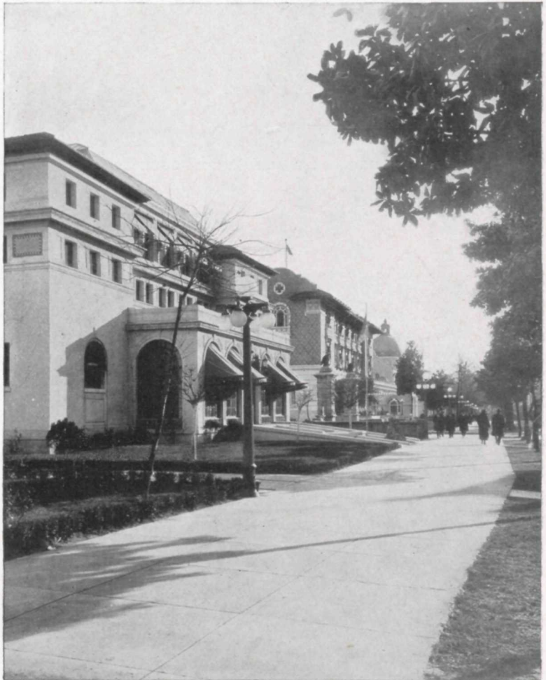
Bathhouse Row Facing Central Avenue
