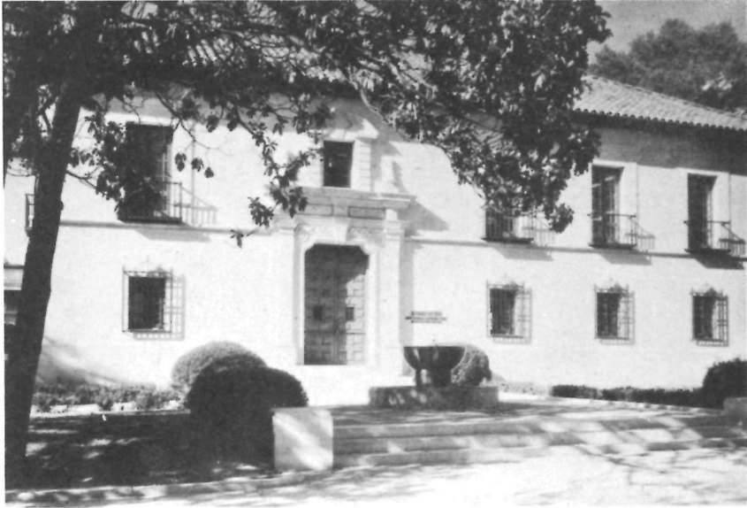
NEW ADMINISTRATION BUILDING
