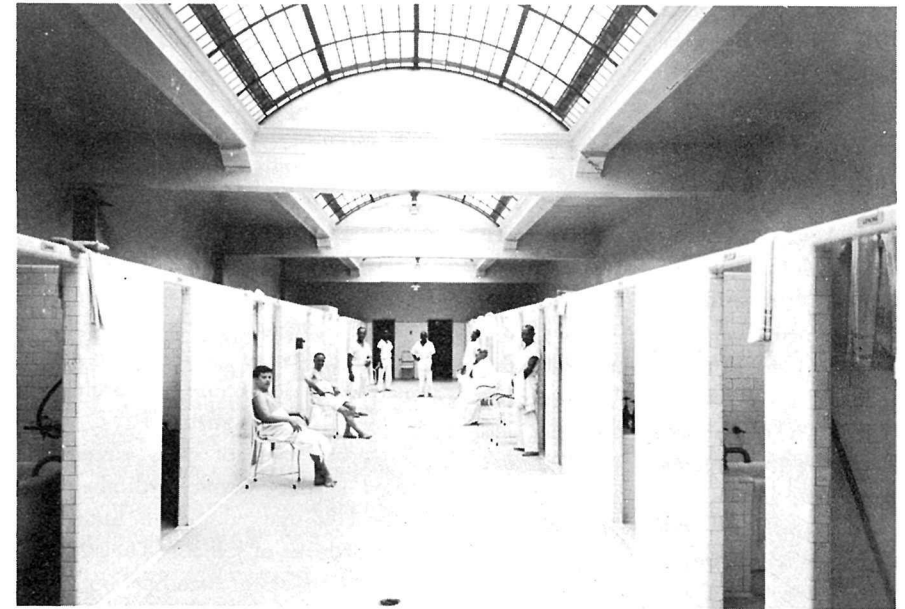
INTERIOR OF BATHHOUSE
