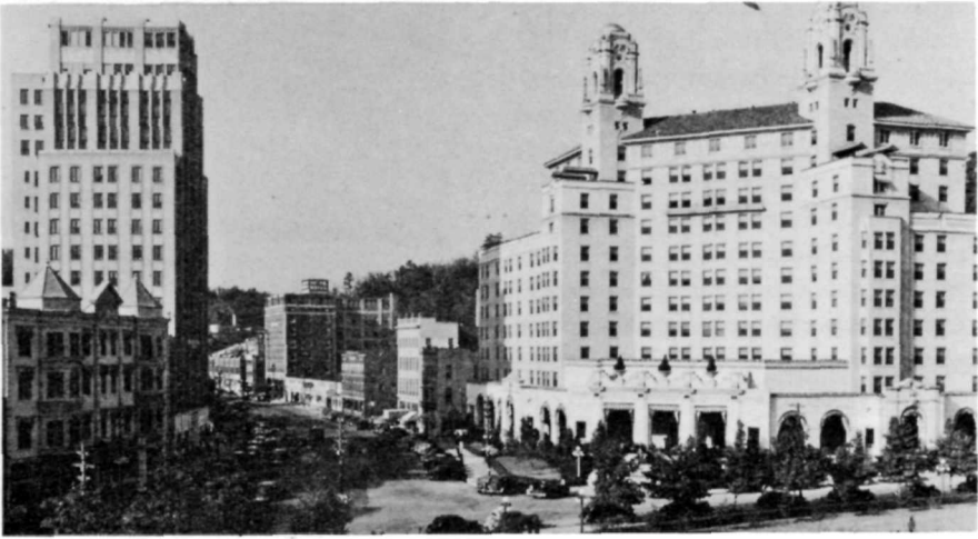
CENTRAL AVENUE, CITY OF HOT SPRINGS
