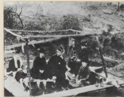
The earliest bathhouses (above) were crude structures of canvas and lumber, little more than tents, that perched over individual springs or reservoirs carved out of the rock. Later, timber structures, which were subject
