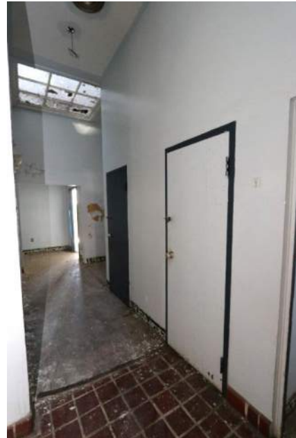
XAI.85 – Hallway 222. Looking southwest.
