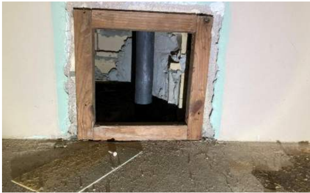
XAI.71 – Closet 213. Utility access at base of wall.
