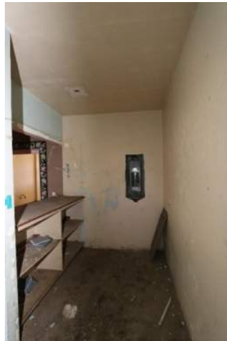
XE.27 Removed Dead Front
