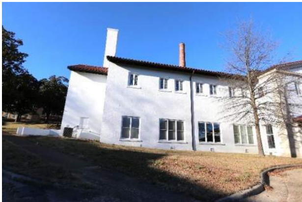
XAE.5 – South face of the building, west end.
