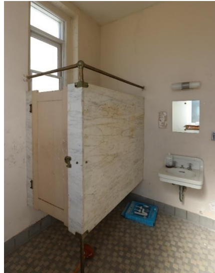
XAI.9 – Toilet 104. Historic marble partition.
