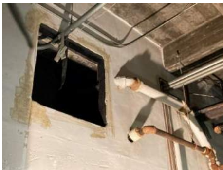
XAI.27 – Mechanical 114. Hole cut into wall.
