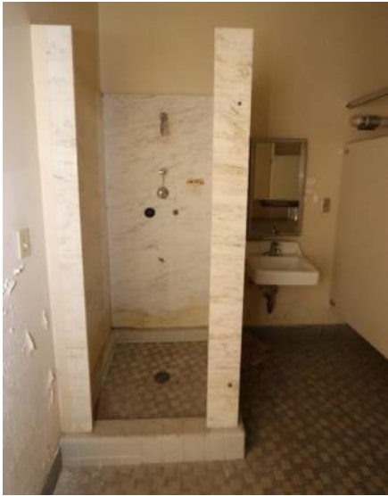
XAI.12 – Toilet 105. Marble shower partition.
