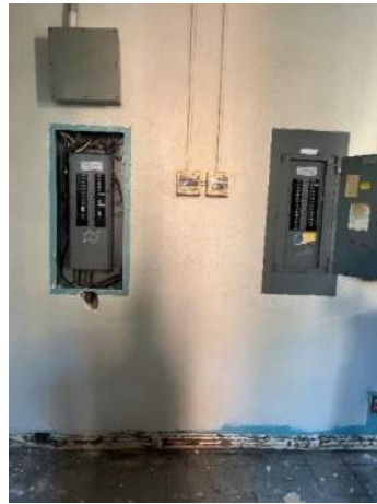
XE.26 Removed Dead Front
