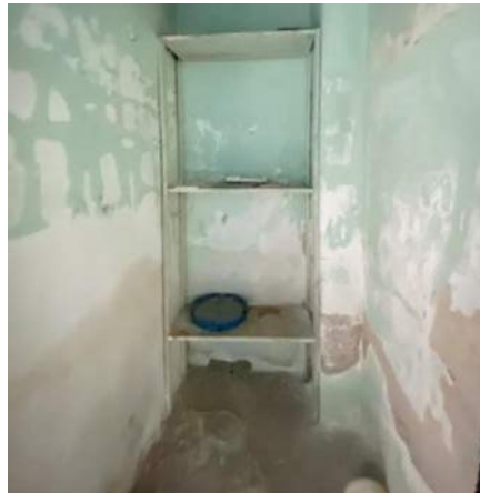
XAI.54 – Closet 204. Looking south.
