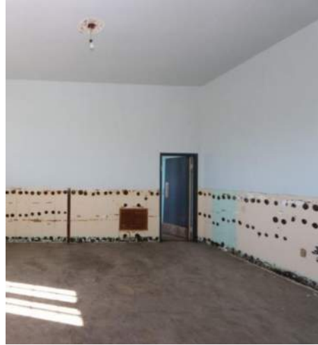
XAI.60 – Room 207. Looking northwest.
