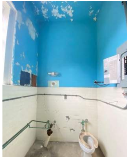
XAI.56 – Toilet 205. Looking south.
