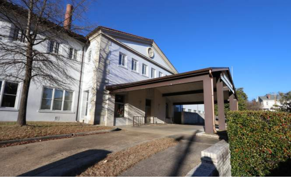
Libbey Memorial PMC, Exterior South Elevation (STRATA, 2022)
