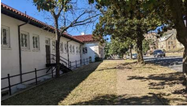
XC.1 – Exterior at north lawn, looking west.
