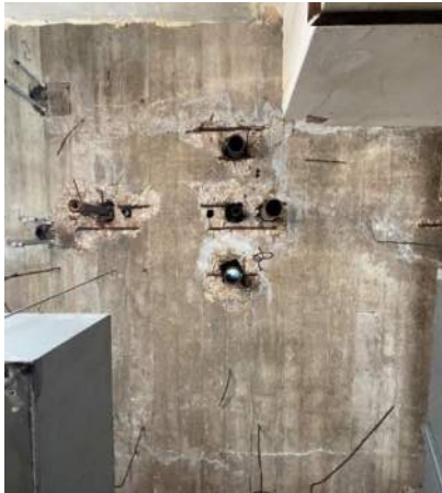
XAI.38 – Mechanical 119. Exposed concrete ceiling.
