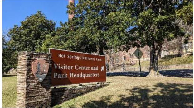
XC.7 – Exterior at south lawn, looking north.
