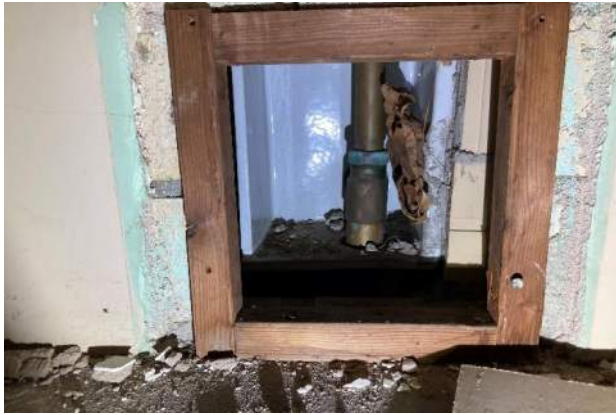
XAI.70 – Closet 212. Utility access at base of wall.
