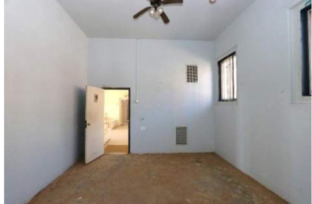
XAI.84 – Locker Room 221. Looking west.
