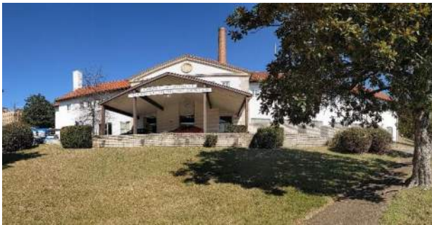
XC.2 – Exterior at south lawn, looking north.
