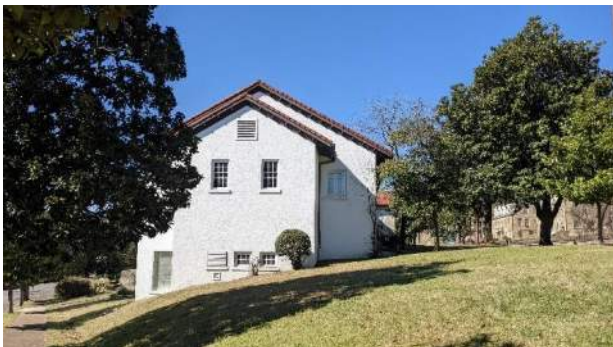
XC.4– Exterior at east lawn, looking west.
