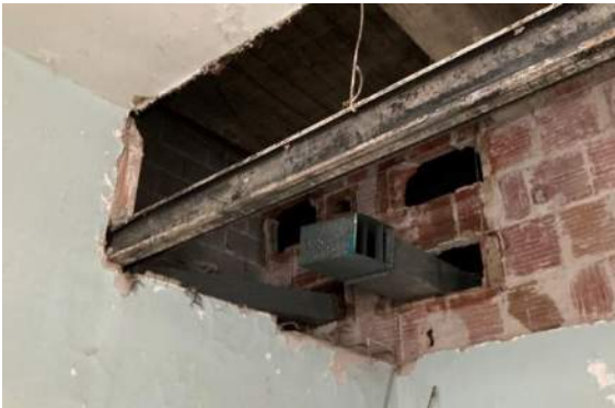
XAI.20 – Office 109. Exposed clay tile wall.
