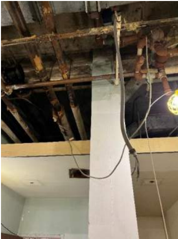
XM.4 Existing Piping
