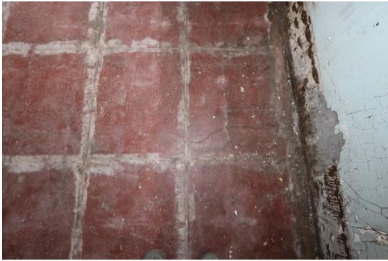
XAI.6 – Office 102. Concrete floor.
