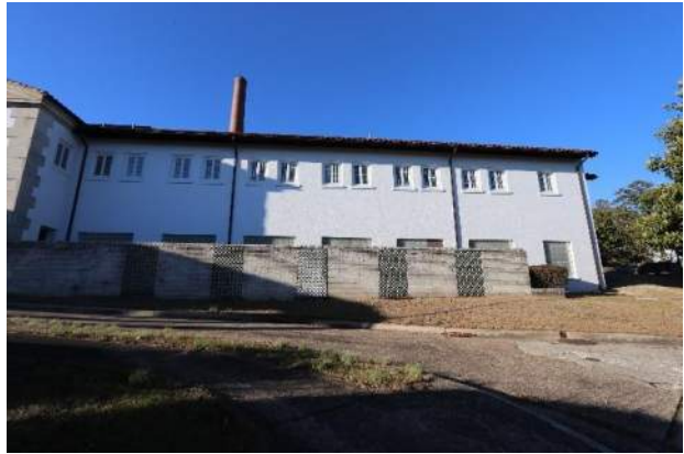
XAE.6 – South face of the building, east end.
