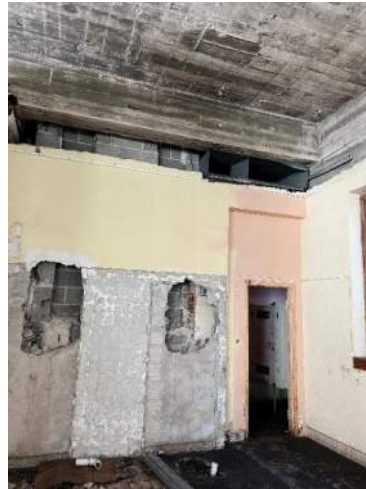
XM.6 Demolded Ductwork
