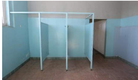
XAI.62 – Locker Room 208. Looking west.
