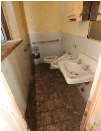
XAI.40 – Toilet 120. Looking east.
