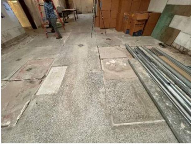
XA.51 – Men's Bath Hall 113. Detail of flooring variations.
