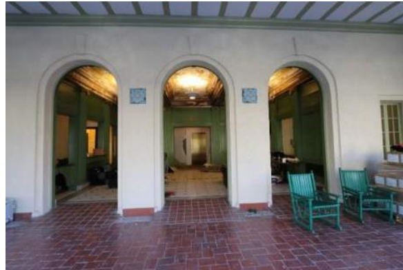
XA.28 – Sunporch 109. Looking east toward Lobby.
