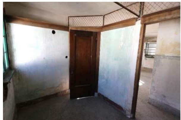
XA.110 – Hall 310. Looking east.
