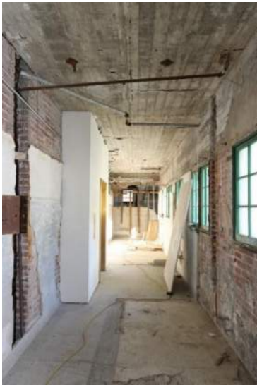
XA.82 – Hall 211. Looking north.
