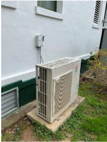
XM.7 Elevator Equipment Room Condensing Unit
