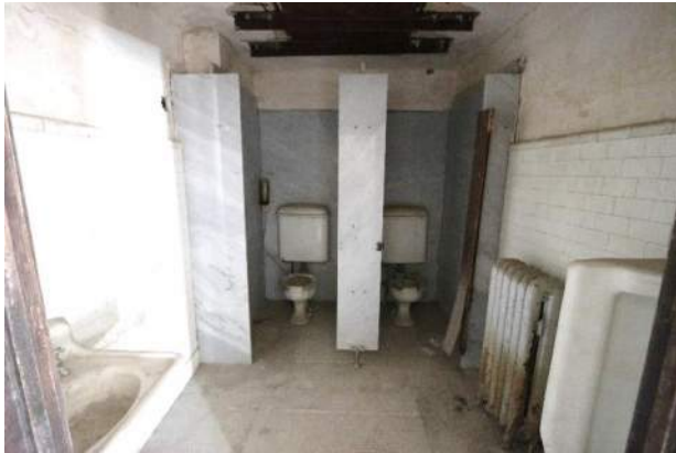
XA.106 – Toilet 308. Looking east.
