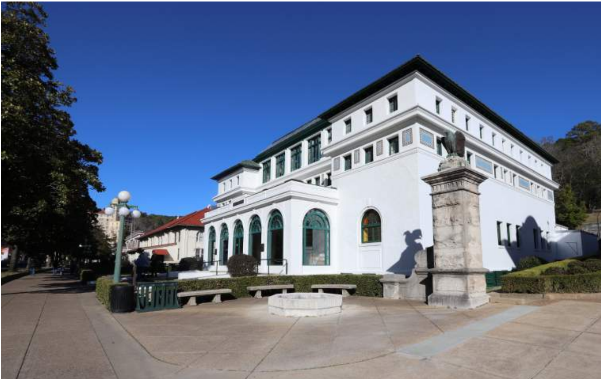
Maurice Bathhouse, Exterior Southwest Corner (STRATA, 2022)
