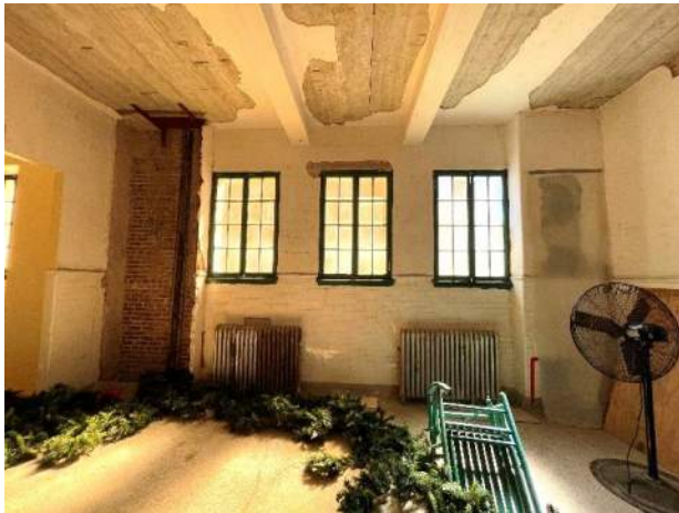
XA.58 – Men's Cool Room 115. Looking South at chases.
