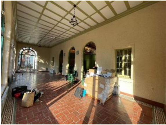
XA.30 – Sunporch 109. Looking north.
