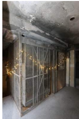
XA.92 – Men's Stair 303. Looking northeast.
