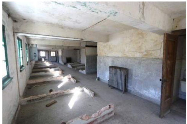
XA.104 – Men's Lounge 306. Looking northwest.
