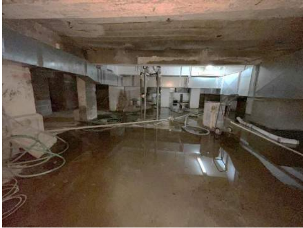
XA.1 – Basement B01 – Typical Conditions.
