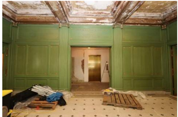
XA.34 – Lobby 110. Lobby, looking east.
