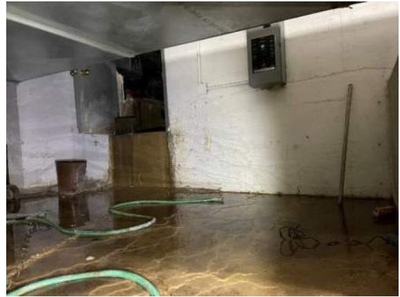
XA.9 – B01 Room with standing hot spring water from crawspace.
