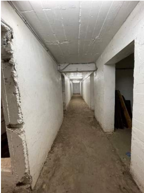
XA.7 – B11 Hall with low overhead beam.
