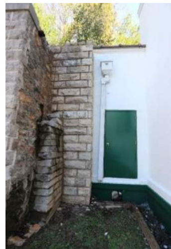
XE.24 Exterior Exit Door
