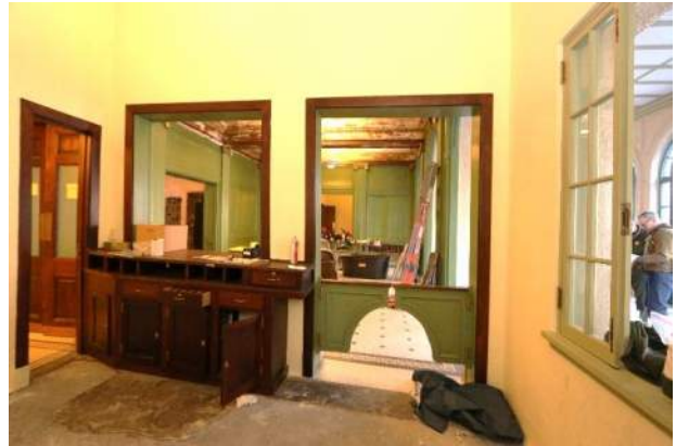
XA.22 – Check-In Office 104. Looking south.
