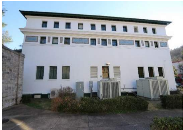
XAE.3 – Exterior. North face of the Maurice with the equipment yard.
