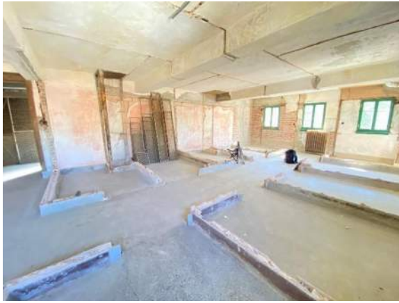
XA.93 – Women's Lounge 304. Looking southwest.
