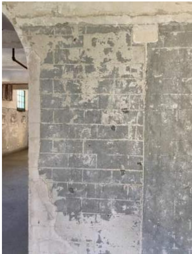
XA.71 – Women's Dressing 203. Detail of faux tile walls.
