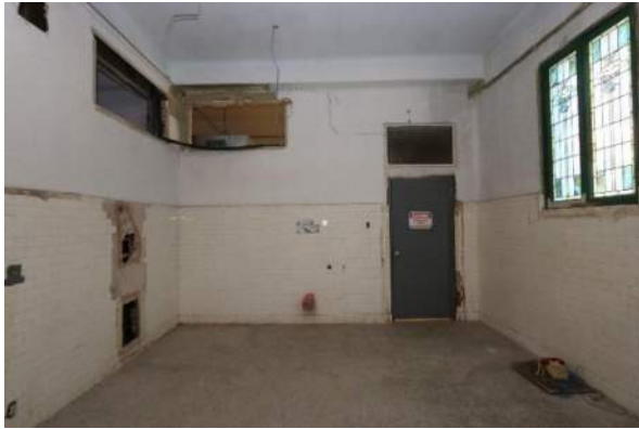
XA.18 – Women's Pack Room 101. Looking west.
