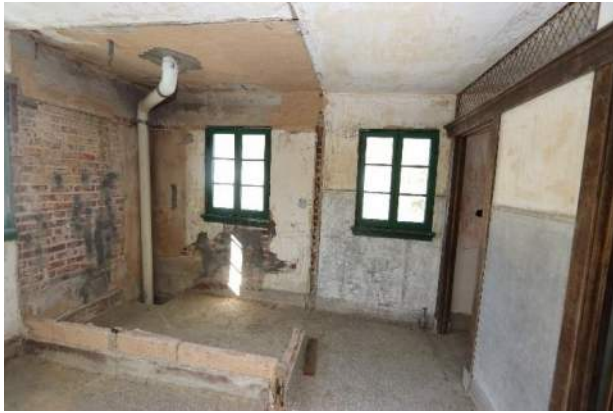
XA.105 – Men's Lounge 306. Looking west.
