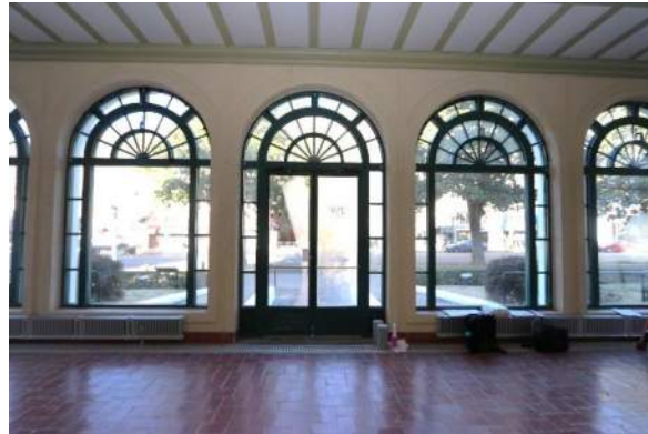
XA.29 – Sunporch 109. Looking west at main entrance.
