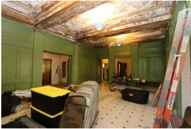
XA.37 – Lobby 110. Lobby, looking southeast.
