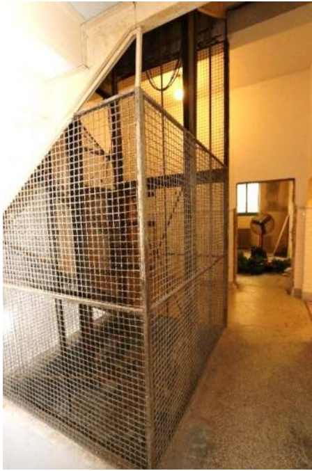
XA.42 – Stair Hall 112B. Original caged elevator.
