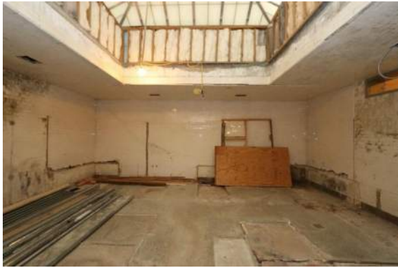
XA.46 – Men's Bath Hall 113. Skylight in Men's Bath Hall, looking south.
