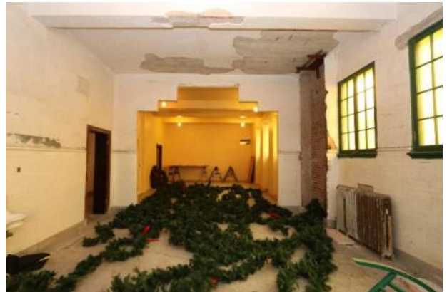
XA.56 – Men's Cool Room 115. Looking east.
