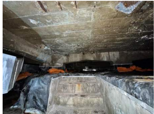
XA.11 – B19 Crawlspace looking east.
