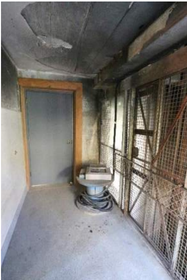
XA.88 – Women's Stair 310. Looking east.
