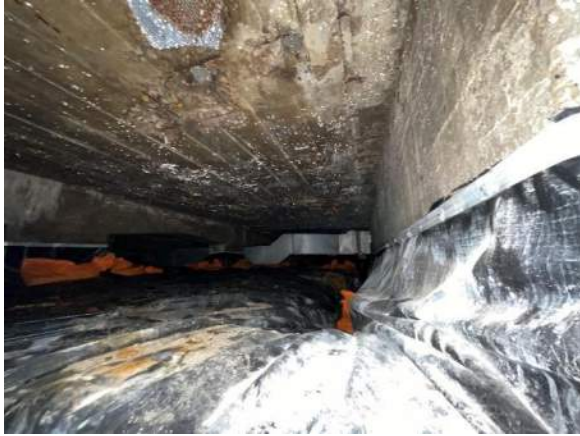
XA.12 – B19 Crawlspace looking south.
