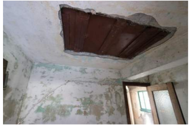
XA.114 – Maurice Office 311. Looking at infilled skylight.
