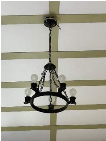
XA.31 – Sunporch 109. Detail of light fixture and ceiling.
