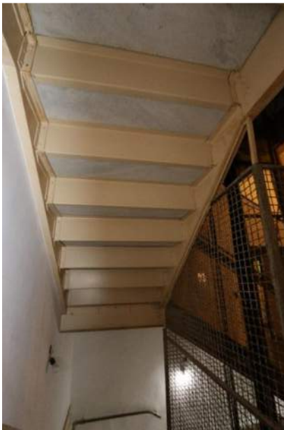
XA.43 – Stair Hall 112B. Original cast iron stairs with marble treads.
