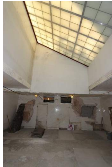
XA.49 – Men's Bath Hall 113. Detail of center skylight.
