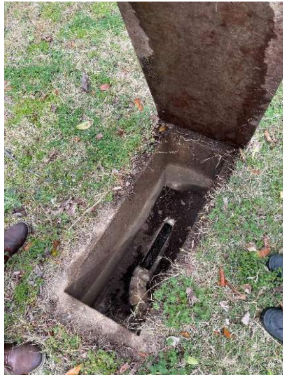
XAE.18 – Access to Display Spring drainage at NE of building.
