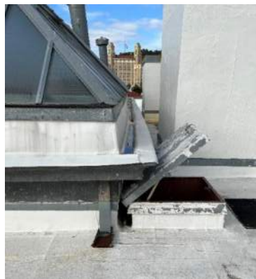
XE.4 Roof Hatch
