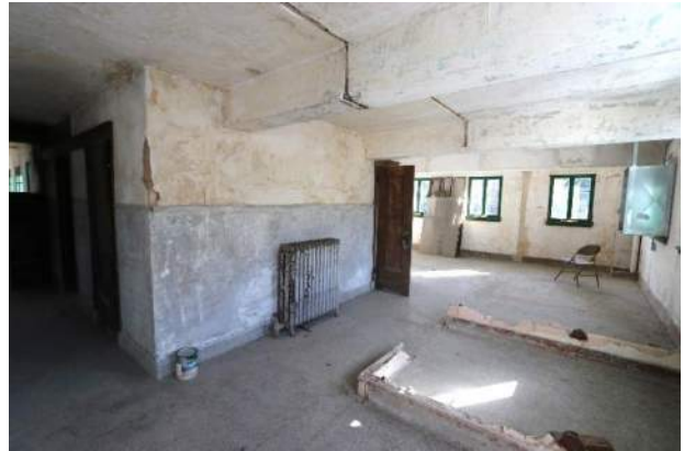
XA.103 – Men's Lounge 306. Looking northeast.
