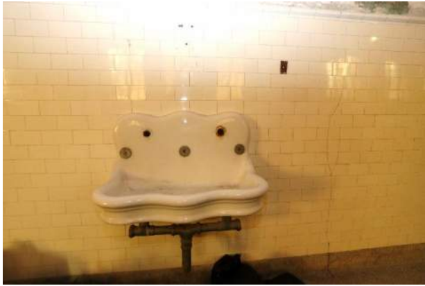
XA.57 – Men's Cool Room 115. Tile wainscoting and sink
