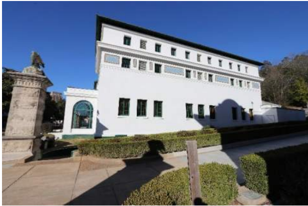
XAE.5 – Exterior. South face of the Maurice from the Promenade.
