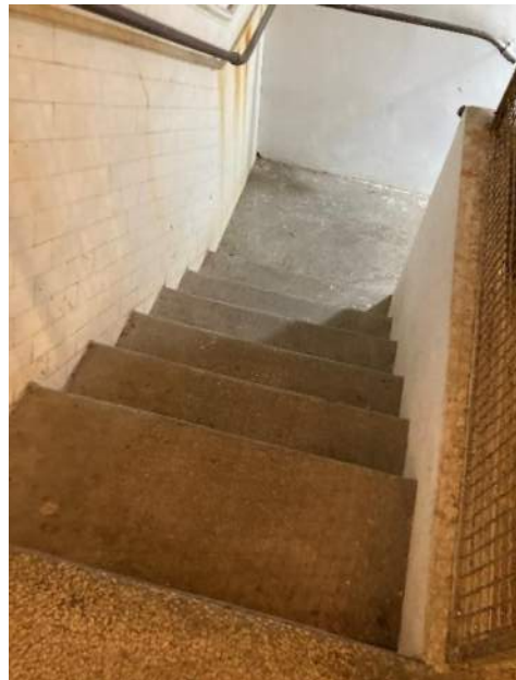
XA.45 – Stair Hall 112B. Concrete stair to basement.
