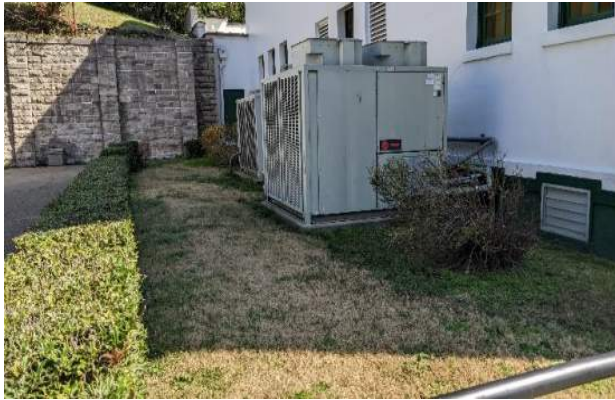
XAE.6 – Exterior. North equipment yard, looking east.
