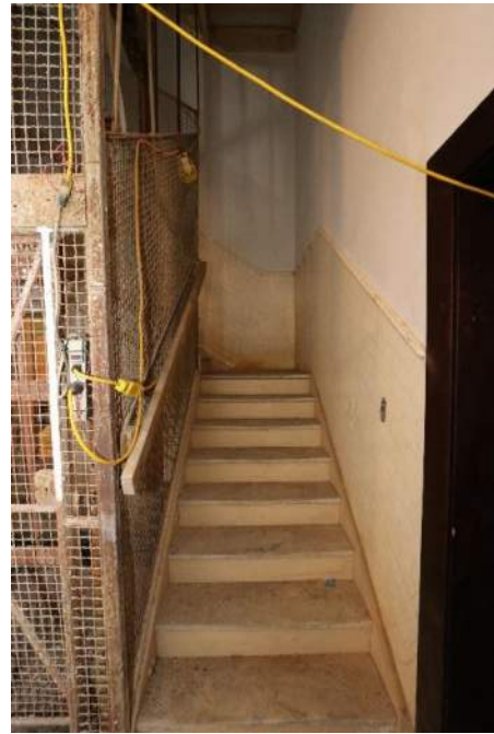
XA.44 – Stair Hall 112B. Original cast iron stairs with marble treads.
