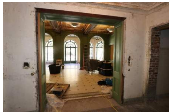
XA.41 – Hall 110E. View from elevator hall into Lobby.
