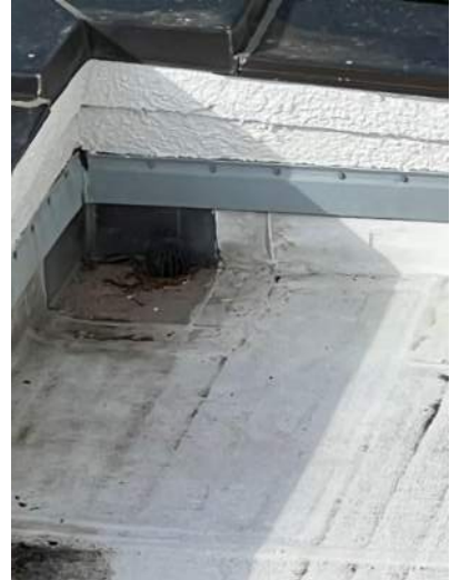
XP.6 Entry Roof Drain
