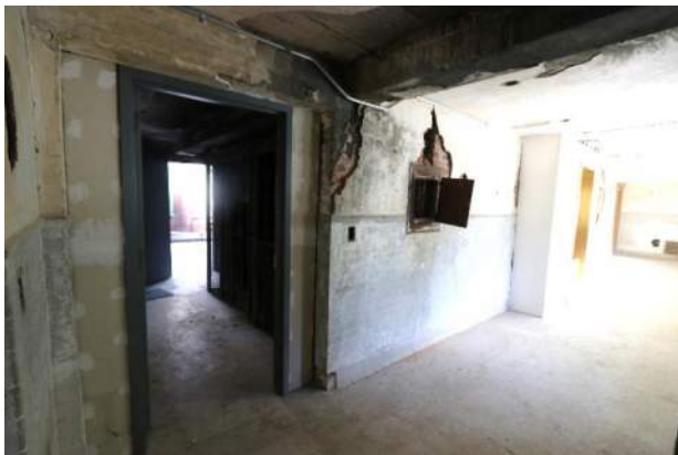
XA.89 – Hall 302. Looking northwest.
