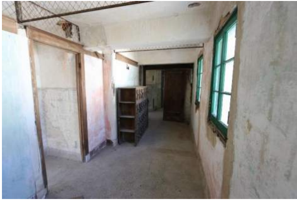
XA.111 – Hall 310. Looking west.
