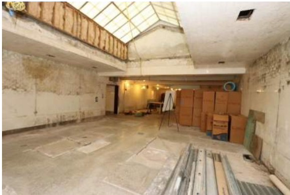
XA.47 – Men's Bath Hall 113. Skylight in Men's Bath Hall, looking north.
