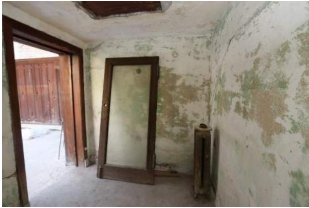
XA.112 – Maurice Office 311. Looking west.
