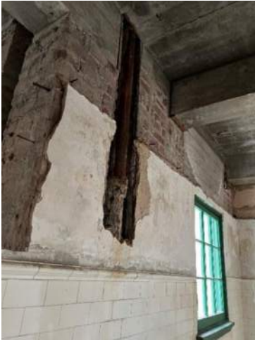
XP.8 Existing Waste Piping
