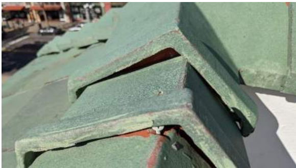
XAE.21 – Roof. Parapet clay cap tile.
