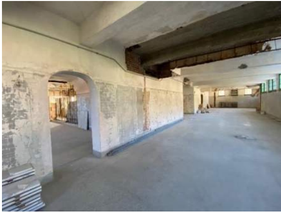
XA.70 – Women's Cool Room. Looking southeast.
