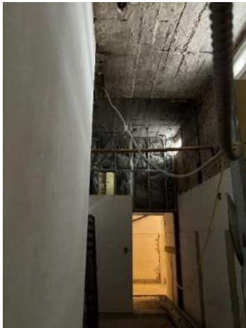
XE.35 Support Wiring
