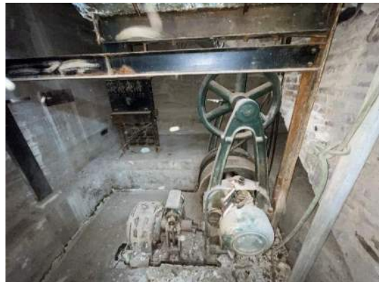
XA.6 – Elevator Pit. Typical historic elevator pit.
