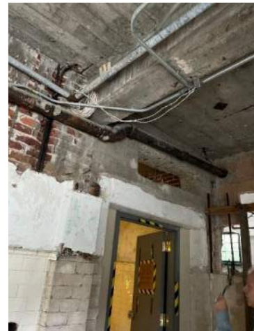
XE.33 Support Wiring
