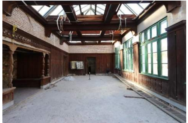
XA.85 – Roycroft Den 300. Looking south.
