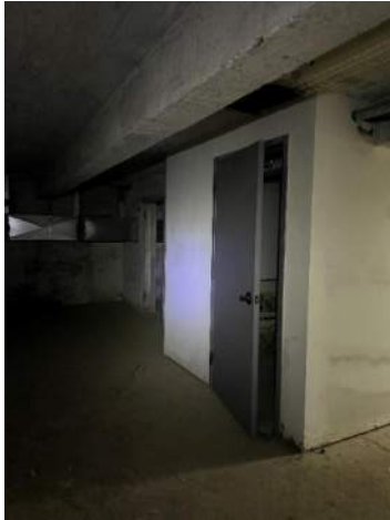
XE.25 Elevator Equipment Entry Door
