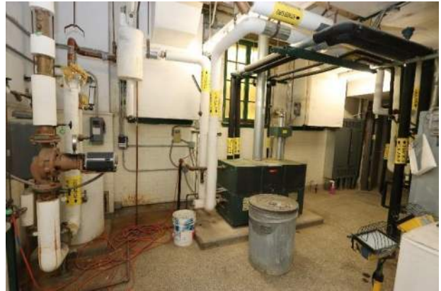
XA.21 – Mechanical 103. Looking north.
