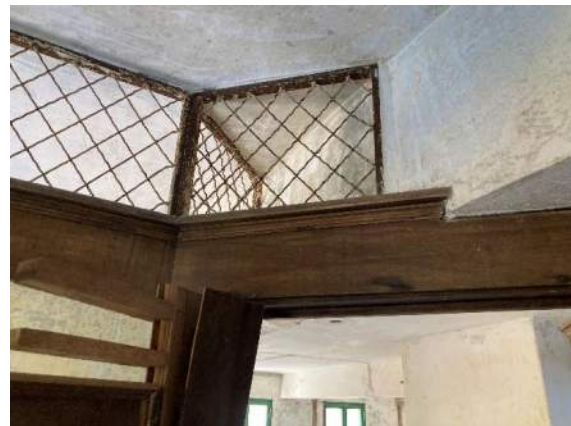
XA.109 – Dressing Rom 309. Looking south at detail at top of wall.
