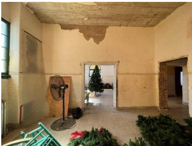
XA.59 – Men's Cool Room 115. Looking west toward Room 116.
