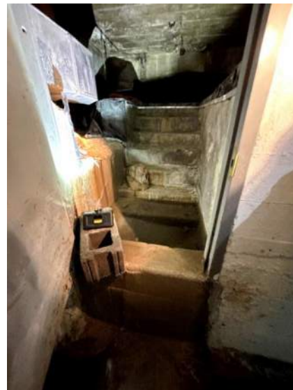
XA.10 – B19 Steps into crawlspace with hot spring.
