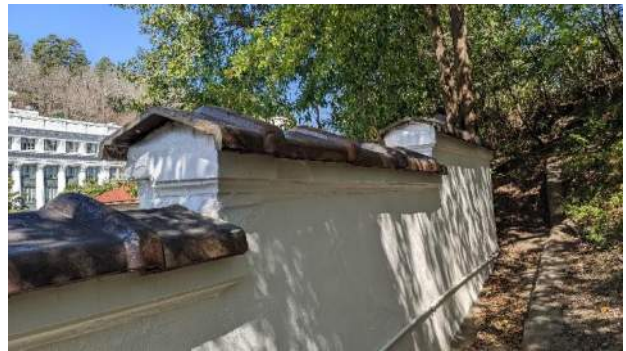
XAE.24 – Roof parapet with clay tiles at east wall, northeast roof.
