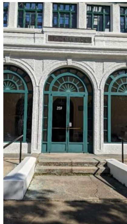
XAE.10 – Sunporch. Damaged stair, window, door.
