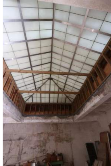
XA.55 – Women's Bath Hall 114. Bath Hall, Skylight, looking north.
