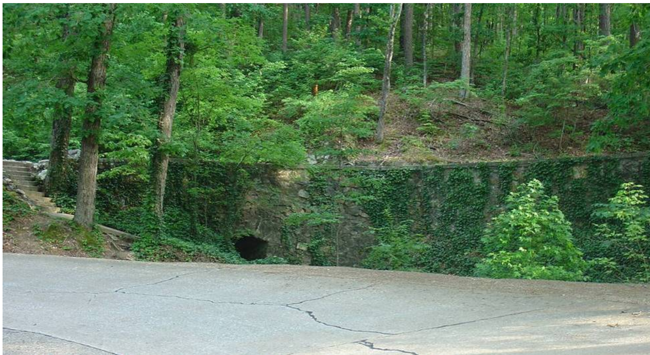
Mortared Stone Retaining Wall with Culvert (Hot Springs Mountain) (CLR 2010, III-113, Figure 3-185)
