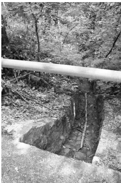
Mortared Stone Spillway on Oak Trail (West Mountain) (CLR 2010, III-132, Figure 3-232)
