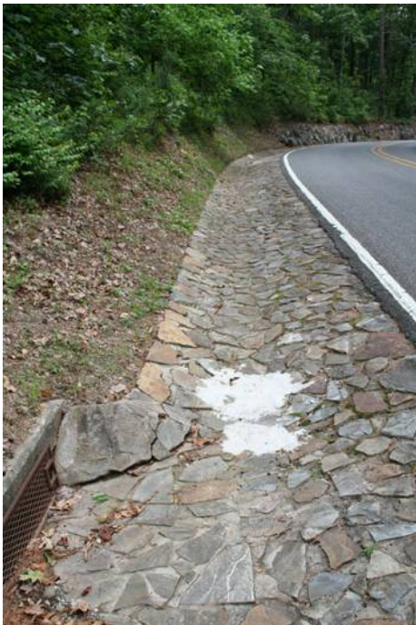
Mortared Stone Gutter at Road (West Mountain) (CLR 2010, III-125, Figure 3-211)
