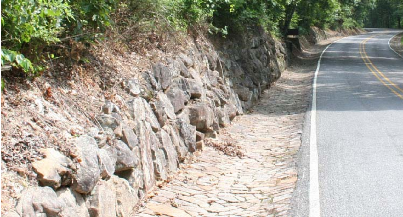
Stone Retaining Wall at Road (West Mountain) (CLR 2010, III-125, Figure 3-210)
