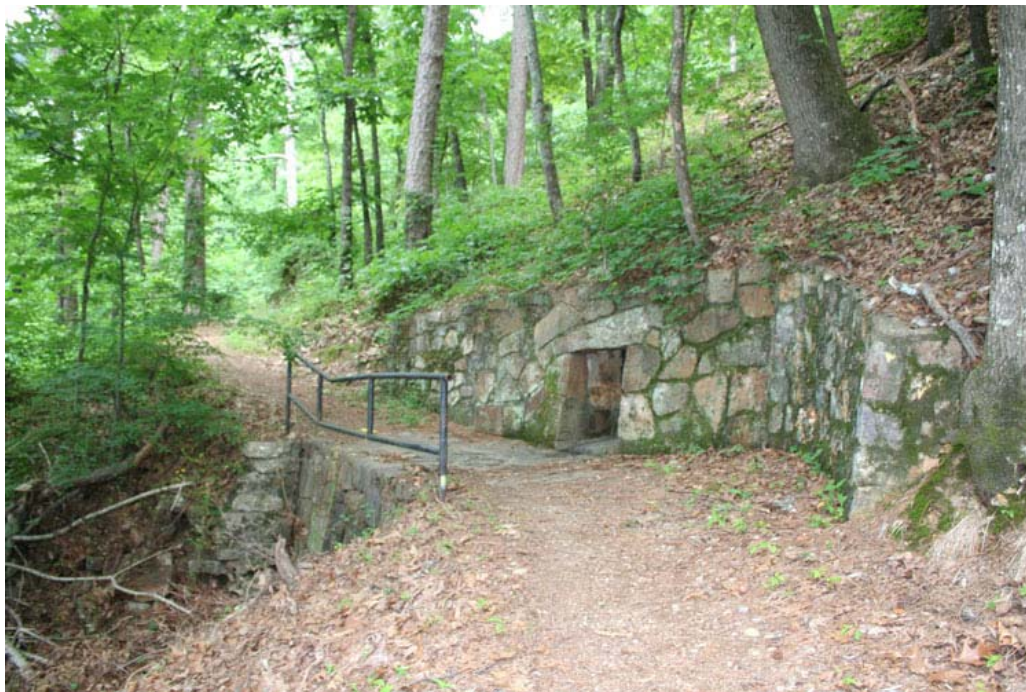
Mortared Stone Bridge/Culvert at Oak Trail (West Mountain) (CLR 2010, III-131, Figure 3-231)
