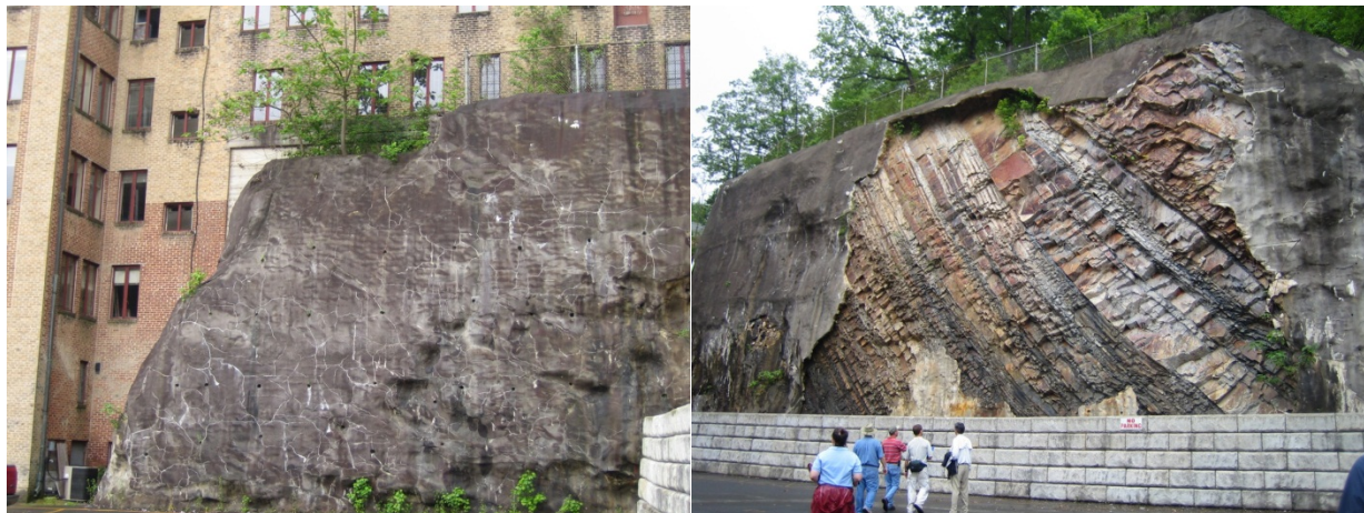
Figure 21. Slope movement mitigation measures. Concrete sprayed against bedrock with drains installed is one type of structure to keep spalling rocks in place on steep slopes. These systems have largely failed due to seeping water undermining the integrity of the concrete, which then dissolves and fractures (left image) from the outside in, becoming a falling hazard itself (right image). Photographs by Trista Thornberry-Ehrlich (Colorado State University), taken in 2007 from a parking lot adjacent to the old Medical Arts building across Central Avenue from the Arlington Hotel.
