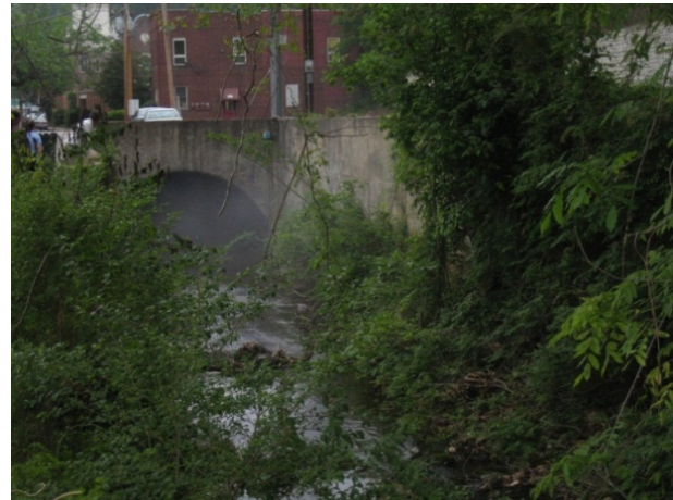
Figure 22. Creek Arch over Hot Springs Creek. The structure channels stream and spring flow beneath the gap between West and North Mountain and Bathhouse Row. The system cannot handle very high flows and floods. Ten hot springs drain into the creek causing steam at the end of the arch. Photograph by Trista Thornberry-Ehrlich (Colorado State University), taken in 2007.
