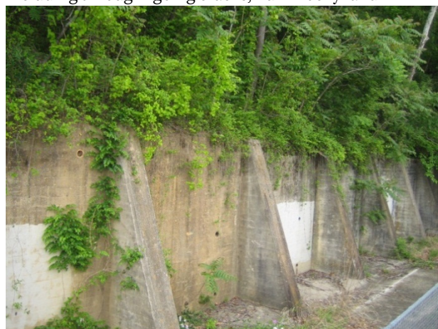
Figure 20. Retaining wall. Structures are placed at the bases of slopes whose toes were excavated to make more room in the narrow valley in the early history of Hot Springs, Arkansas. Photograph by Trista Thornberry-Ehrlich (Colorado State University), taken in 2007.
