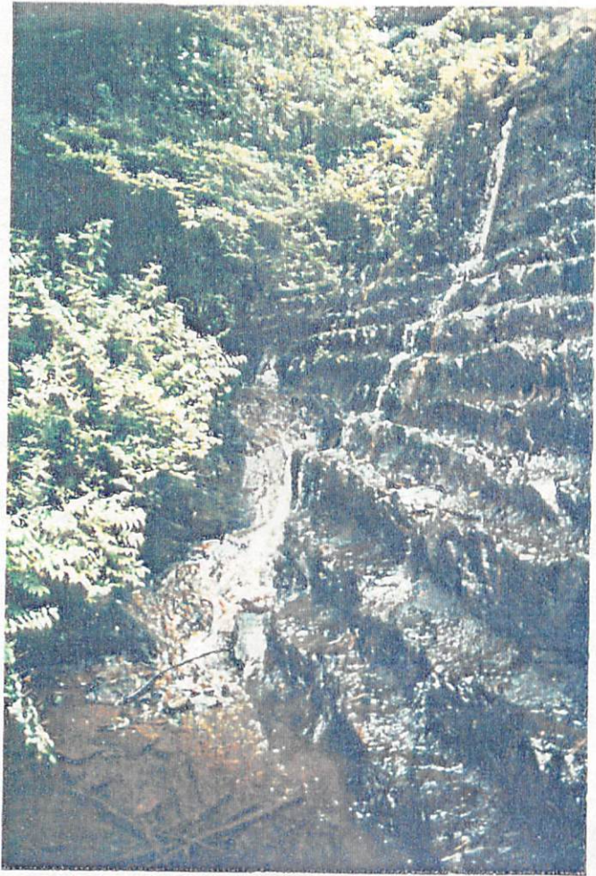
Photo CE-3. Ricks Estate Dam - View of right portion of downstream face and groin from toe of dam. 6-10-82
