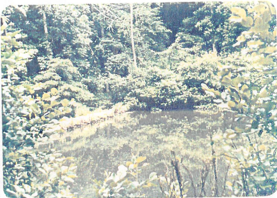
Photo EG-4. Ricks Estate Dam - View of upstream right abutment. 6-10-82
