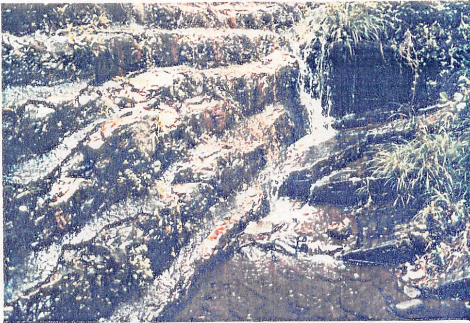
Photo CE-9. Ricks Estate Dam - Closeup of downstream face near left abutment. 6-10-82
