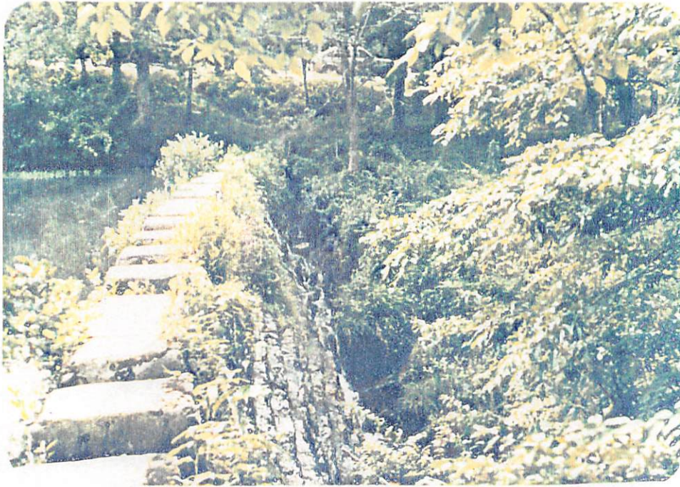
Photo EG-1. Ricks Estate Dam - View of overflow crest. 6-10-82
