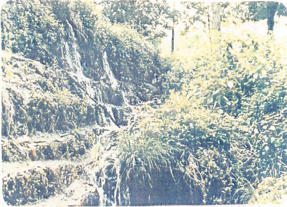
Photo EG-3. Ricks Estate Dam - View of downstream left abutment. 6-10-82
