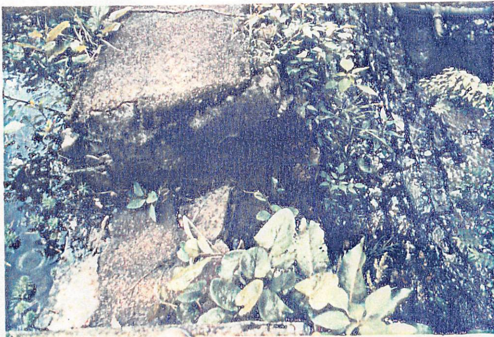
Photo CE-10. Ricks Estate Dam - Closeup of area on crest where stone has been lost from rubble masonry matrix. 6-10-82
