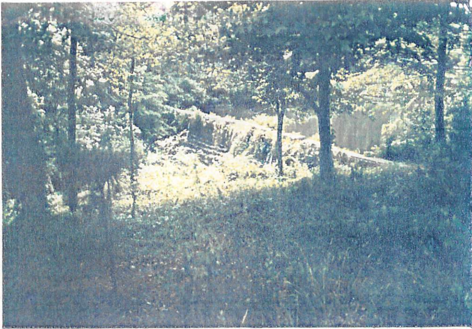
Photo CE-1. Ricks Estate Dam - View of dam from downstream left abutment. 6-10-82
