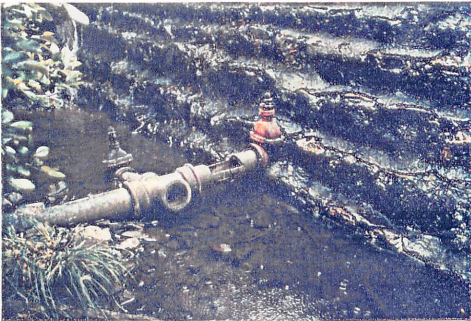
Photo CE-12. Ricks Estate Dam - Outlet works components exposed at downstream toe of dam. 6-10-82
