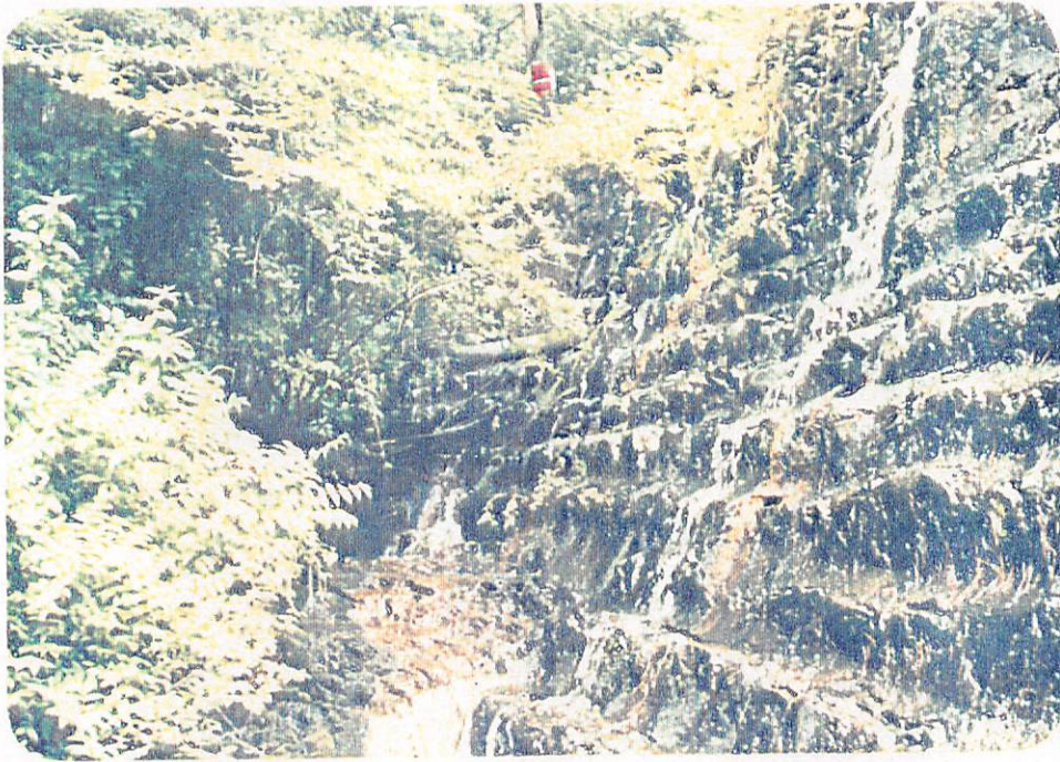
Photo EG-5. Ricks Estate Dam - View of downstream right abutment. .6-10-82
