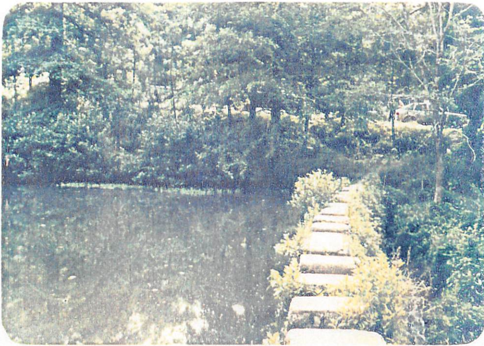
Photo EG-2. Ricks Estate Dam - View of upstream left abutment. 6-10-82
