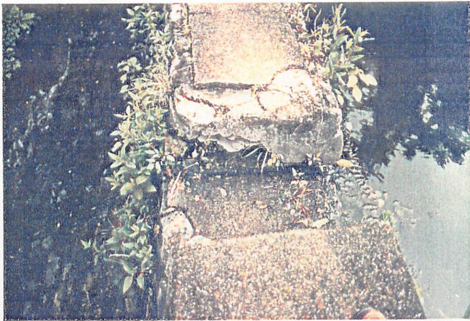
Photo CE-8. Ricks Estate Dam - Closeup view of section of crest. 6-10-82
