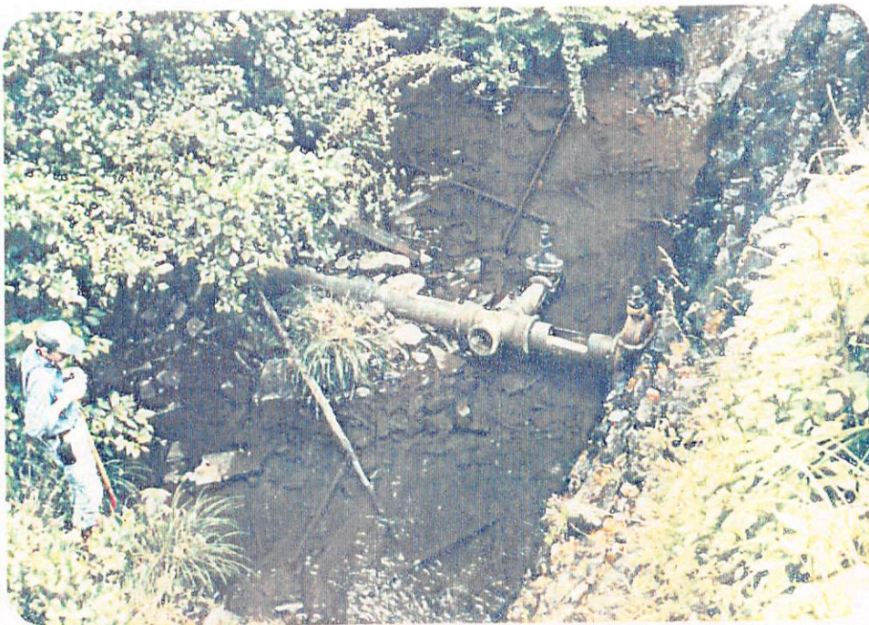
Photo EG-6. Ricks Estate Dam - View of outlet works gate and 8-inch cast iron discharge pipe. 6-10-82
