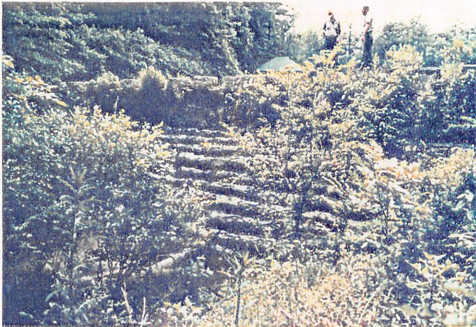
Photo CE-11. Ricks Estate Dam - Downstream face of dam. 6-10-82
