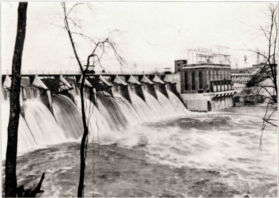
Remmel Dam—First of three hydro-electric power dams on Ouachita River near Hot Springs National Park
