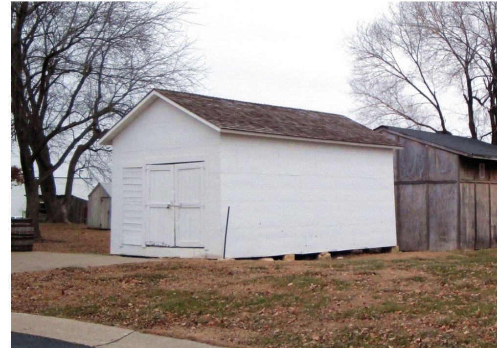
Truman Farm Garage, southwest elevation (Jackson/NPS 2009).
