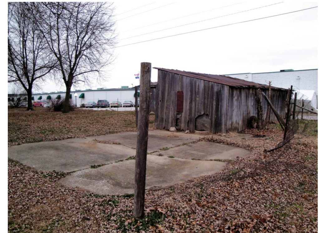
Truman Farm Poultry House, southeast elevation (Jackson/NPS 2009).
