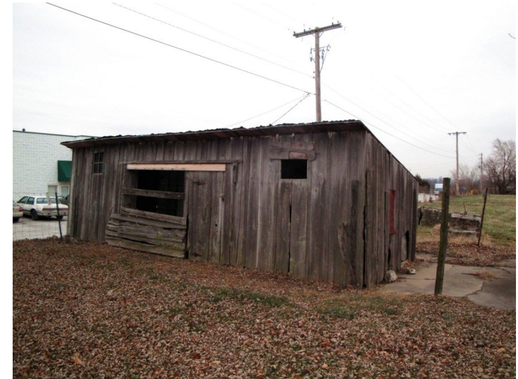
Truman Farm Poultry House, southwest elevation (Jackson/NPS 2009).
