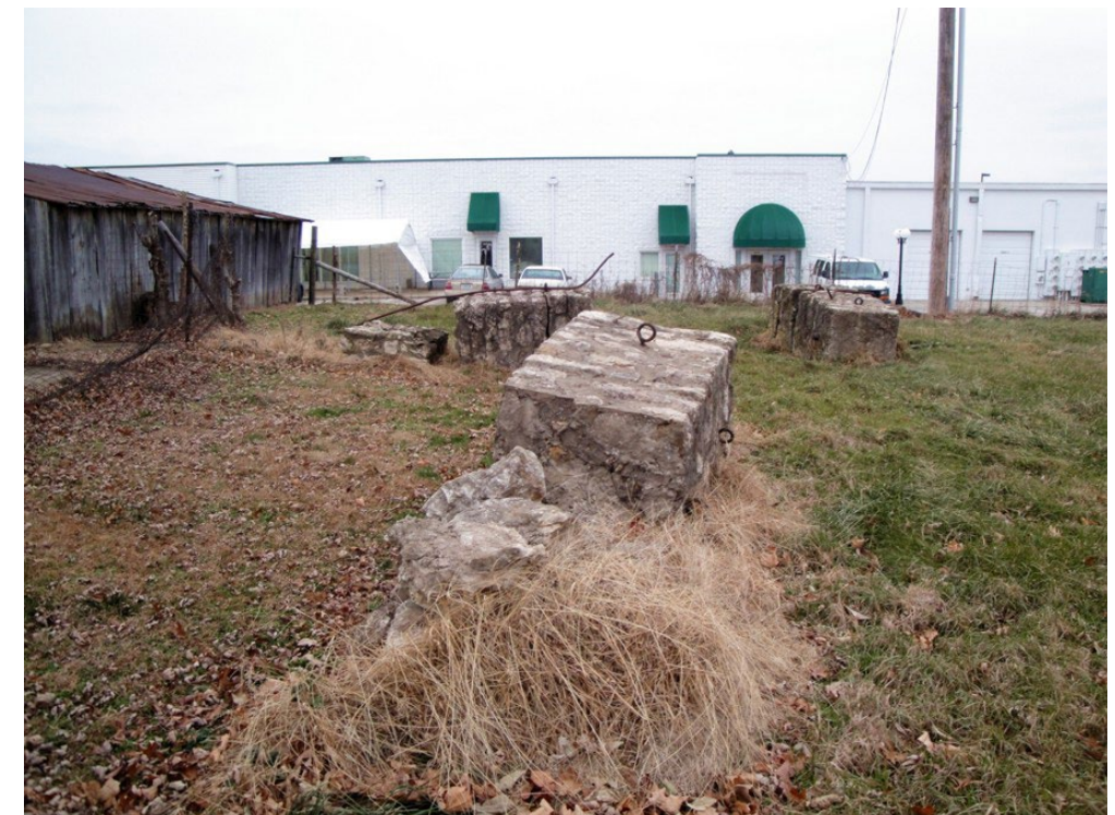
Displaced stone posts located behind the poultry house (Jackson/NPS 2009).
