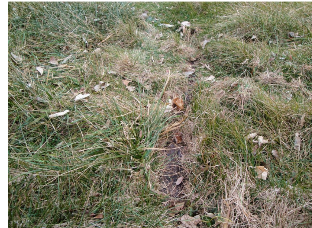
A visible wood threshold to the barn foundation (Jackson/NPS 2009).
