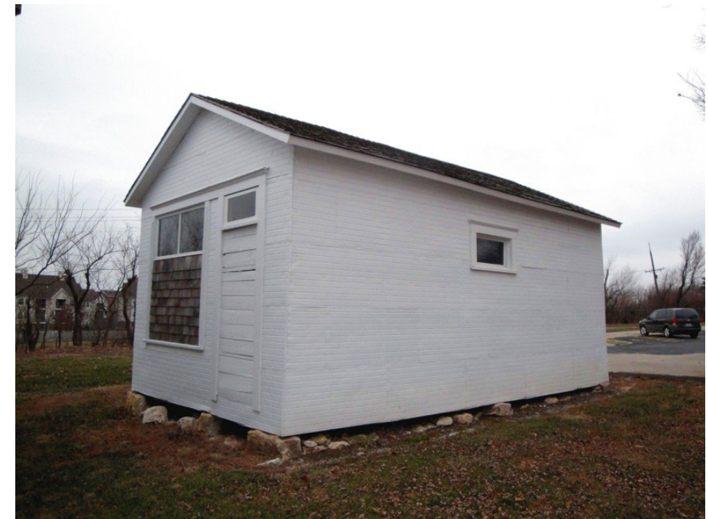
Truman Farm Garage, northeast elevation (Jackson/NPS 2009).
