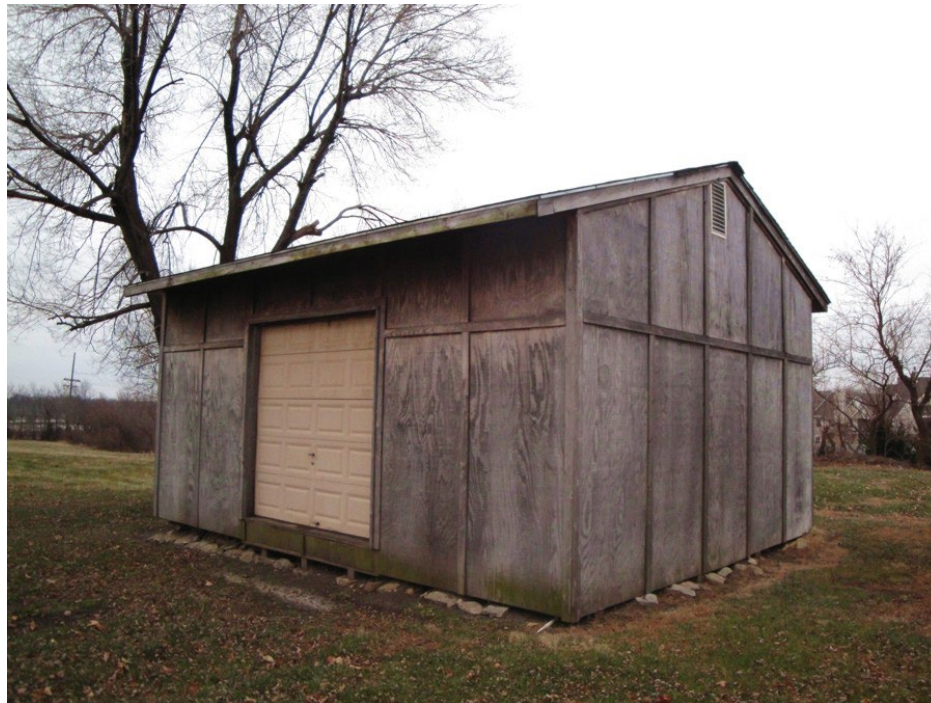
Truman Farm Maintenance Shed, northwest elevation (Jackson/NPS 2009).
