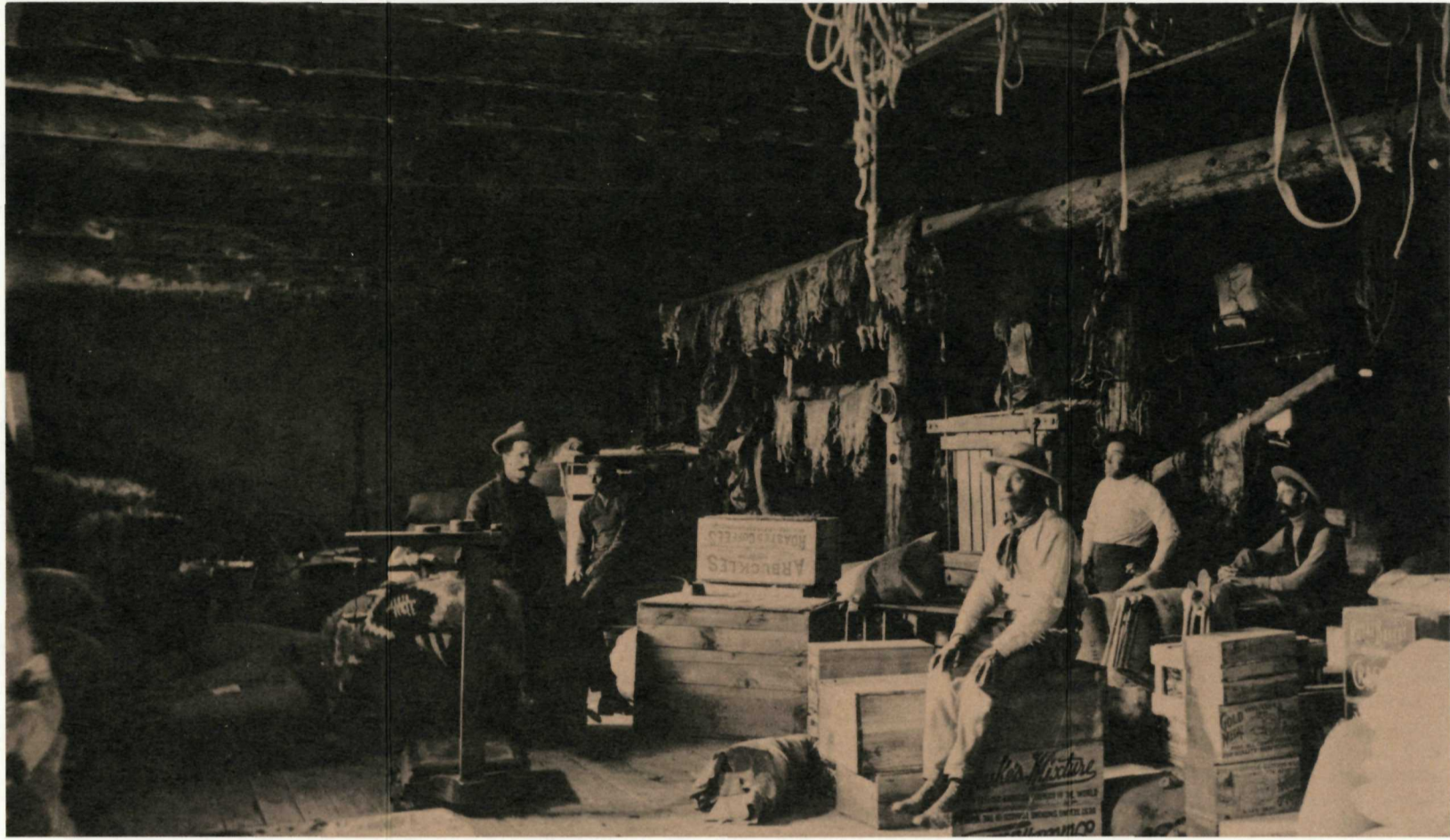
Among goods stored in the warehousing were tobacco, coffee, crackers, ax handles, blankets, harnesses, and pelts.
