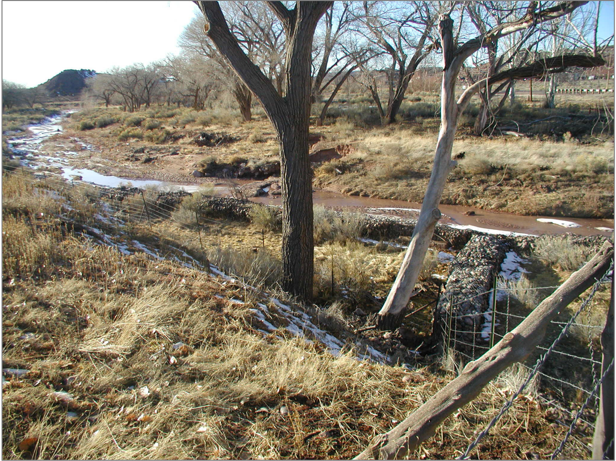
Figure 18. Photograph of Pueblo Colorado Wash. The photograph provides a sense of Pueblo Colorado Wash and its floodplain in the historic site. Hubbell Hill is in the background. Note the gabions (bundles of rocks) that line the nearside of the wash and cut perpendicular toward it. The NPS initially installed gabions in the 1970s. Photograph by Katie KellerLynn (Colorado State University), taken 2007.
