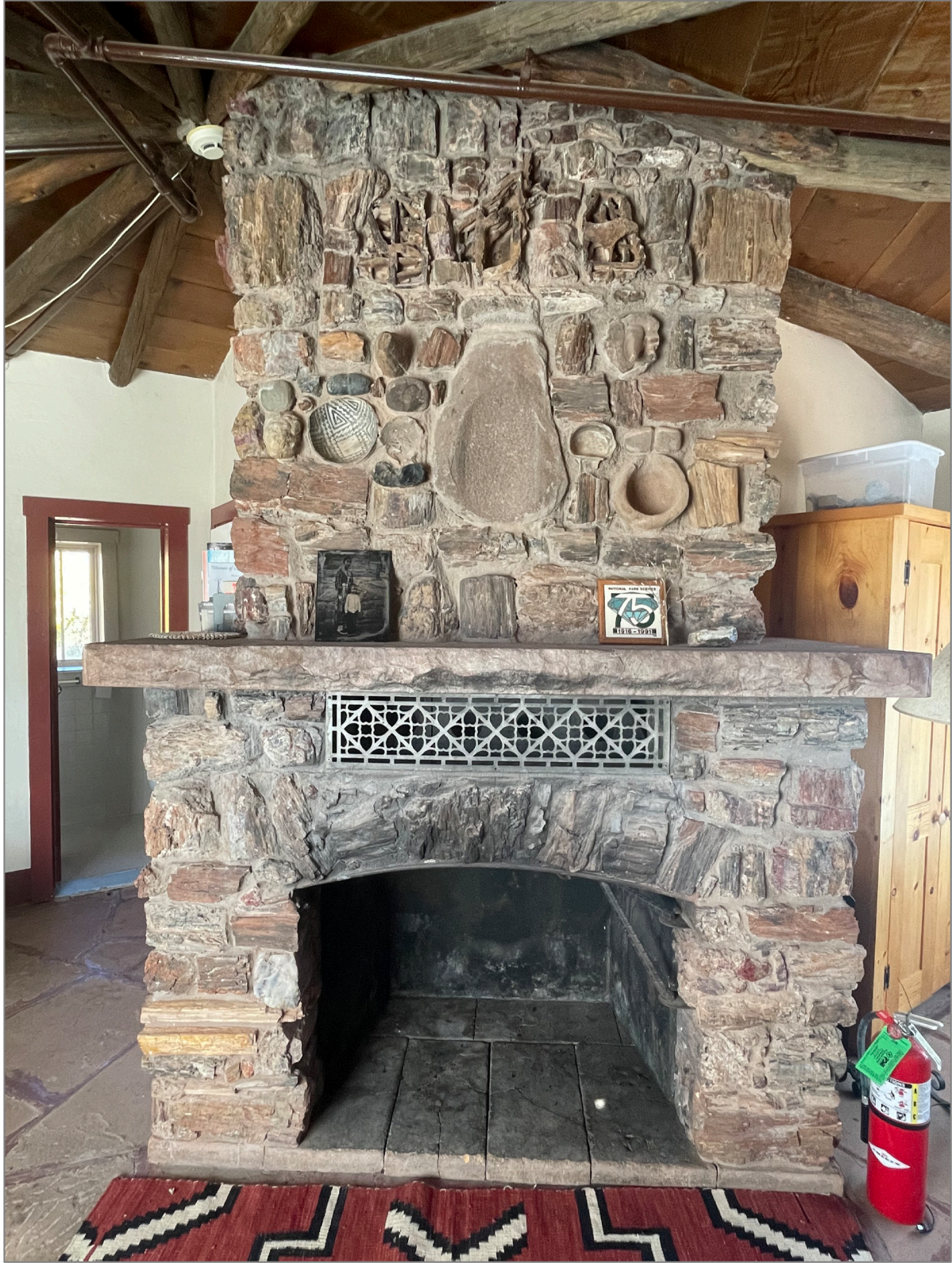
Figure 6. Photograph of fireplace. The massive fireplace in the guest hogan is made of natural stone and petrified wood as well as pottery and other stone items of archeological significance. NPS photograph by Maryann Neubert (Hubbell Trading Post National Historic Site), taken 2023.
