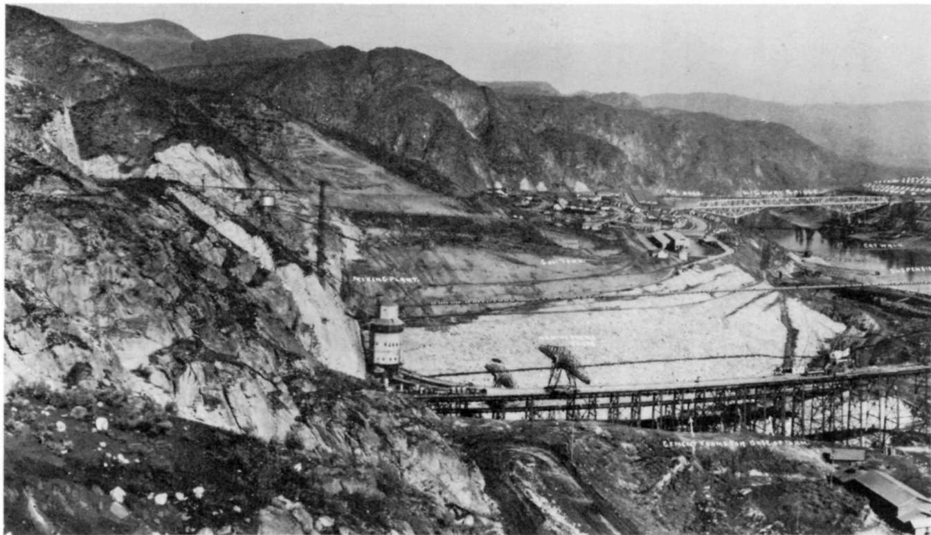
PANORAMIC VIEW OF GRAND COULEE DAM CONSTRUCTION. UPPER PLATE SHOWS WEST SIDE WITH ENGINEERS TOWN IN BACKGROUND. LOWER PLATE SHOWS EAST SIDE CONSTRUCTION WITH MASON CITY IN BACKGROUND.
